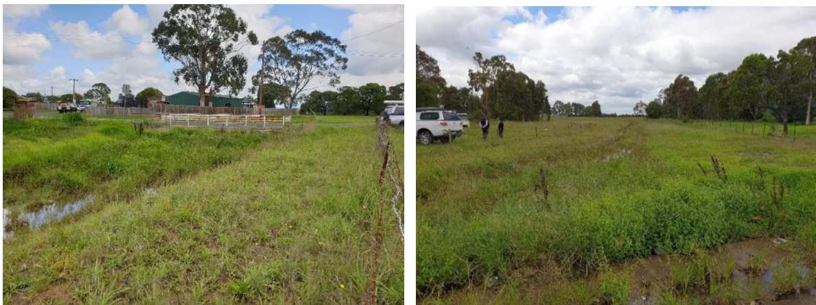
Figure 15. The Landy Street culverts indicating sedimentation and vegetation of the downstream side reducing conveyance (left), and looking east on Landy Street (right)
