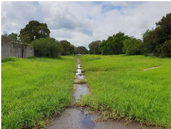
Figure 11. Looking east from Alfred Street at the concrete channel/grassed floodway arrangement
