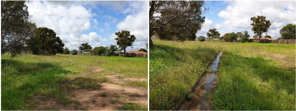
Figure 13. Looking east at Powerscourt Street showing a narrow concrete channel and wide grassed floodway
