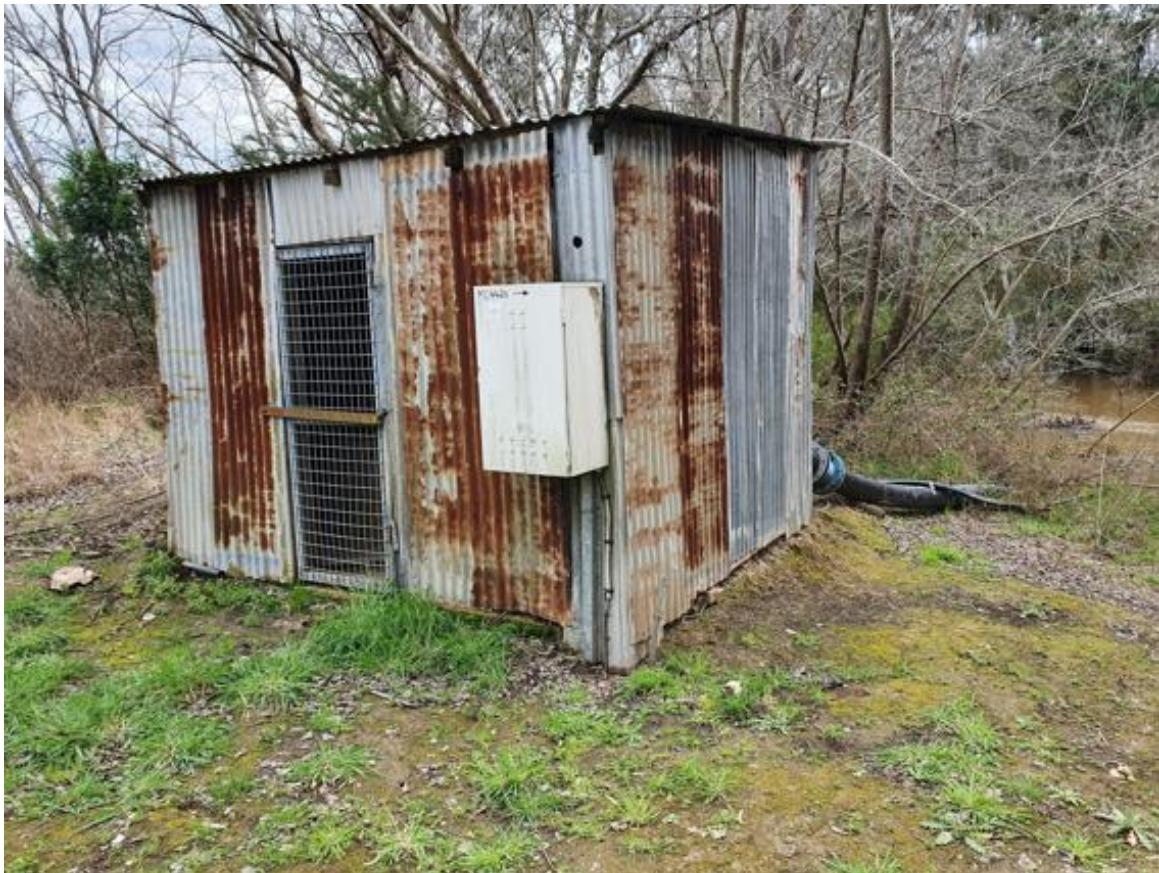
Figure 20: Photo of the pumping station at the Thomson River via which the 550ML water right allows the pumping of water to Kilmany Park Farm via a 250mm underground pipe
