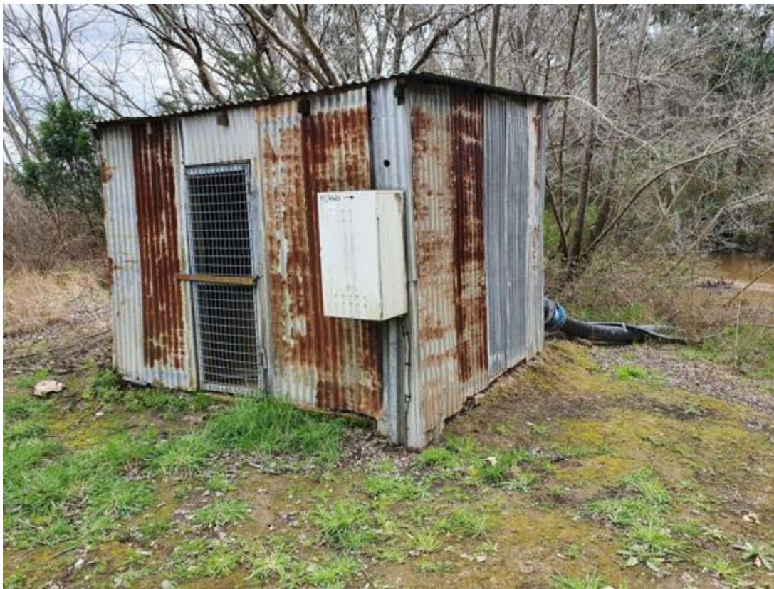
Figure 20: Photo of the pumping station at the Thomson River via which the 550ML water right allows the pumping of water to Kilmany Park Farm via a 250mm underground pipe
