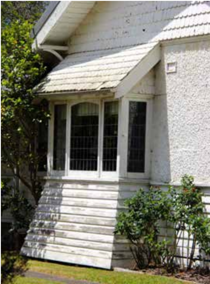
Figure D2. The projecting box window on the west elevation with a detail of the splayed base clad with mitred weatherboards, geometric leadlight timber windows and shingled roof. Half of the base of the exterior walls is timber, with roughcast render to the top half of the wall.
