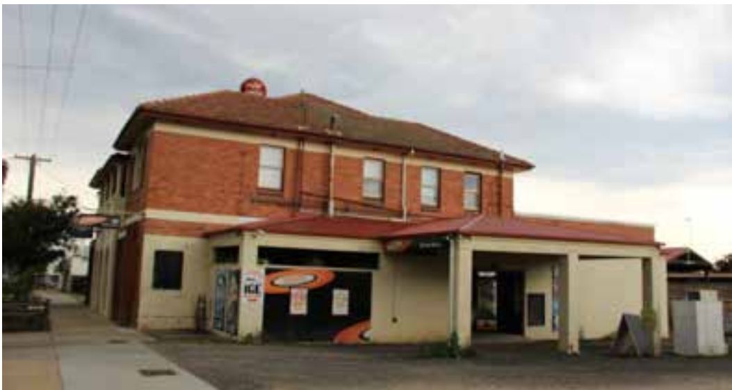
Figure D4. The north elevation has windows in the same style, to the first floor. The ground floor has a modern addition attached, which serves at the drive-through bottle shop.
