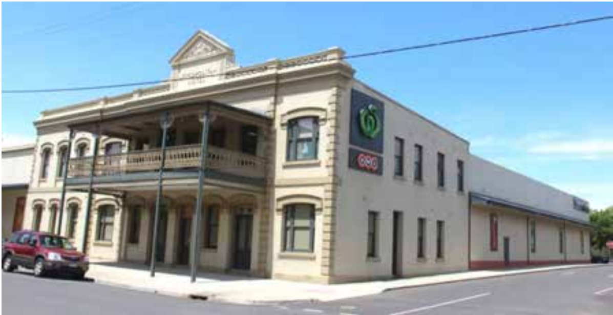
Figure D1. The two-storey building was constructed of brick (overpainted), with tuck pointing to the facade, on a rendered plinth. A decorative parapet to the facade stops at a pediment. The pediment sits central over the two-storey verandah below (reconstructed in 1996).
