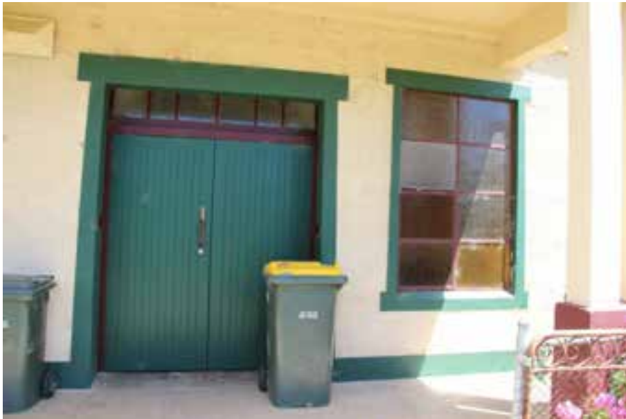
Figure D2. Underneath the porch is an entrance with a pair of wide timber ledged and framed doors with a multipaned metal-framed highlight. The door has a rendered lintel and sides (overpainted); the render to the sides tapers to the tops, giving an Egyptian nuance to the entrance. To the right is a metal-framed 8-paned window of yellow pressed glass, with a rendered sill, lintel and sides, forming a frame to the window.
