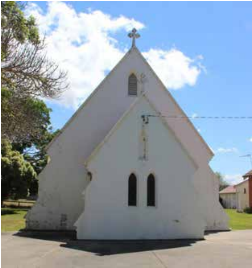
Figure D1. The 1870 church is rendered (overpainted white) and is Victorian Gothic in style. The church has a steeply-pitched gabled roof, parapets to the gabled ends, rendered walls with ruled lines to create an ashlar effect and a central entrance porch.
