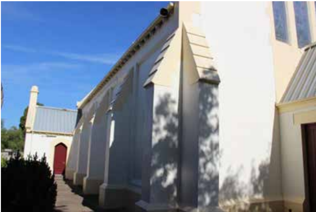
Figure D4. The north elevation has a gabled-roof vestry projecting off the chancel end, with timber ledged door (with a pointed arch opening) facing west. It has a large parapeted gable which appears to extend to form a bellcote.
