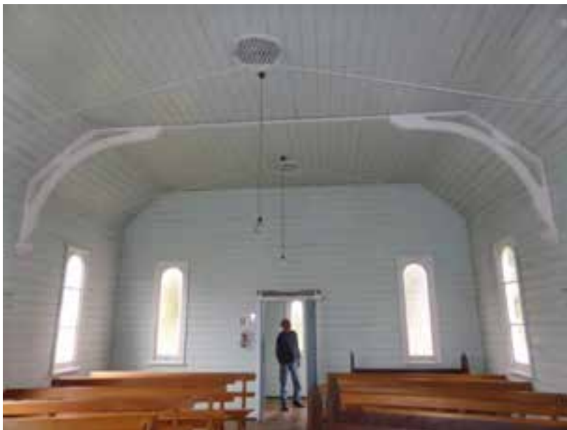
Figure D4. The timber-lined interior of the church with its coved ceiling, metal trusses, decorative metal ceiling vents and decorative timber trusses. (BHG).
