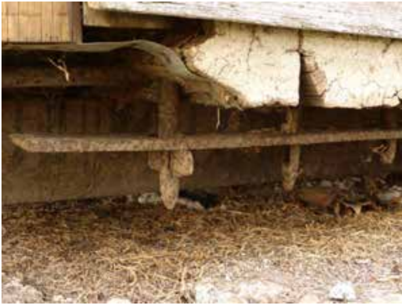
Figure D4. The lock up is constructed of an iron cage clad in timber, making it suitable for prefabrication and easily transported. The ends of the iron rods can be seen at the level below the door.
