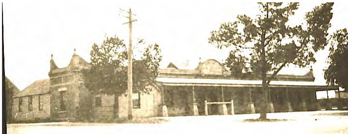
Figure H1. A photo dating to c1930s that showed the facade and west elevation of the hotel (MDHS, ID. P03709VMFF). The facade comprised the parapet with the central pediment. Behind the pediment, the gabled-end of the eastern portion of the building was evident; this gable and hipped roofed building (made of early brick?) behind the 1922 plastered façade is likely to be part of the 1863 building.
