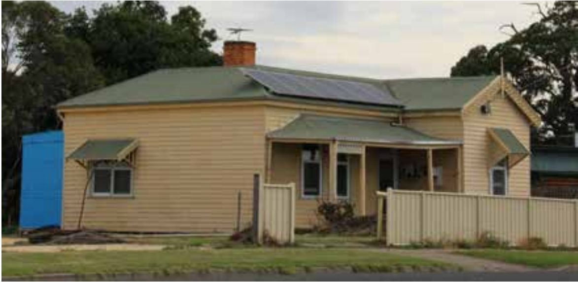
Figure D1. The facade and eastern elevation of the house. The weatherboard house has a shallow-pitched M-hip roof with a projecting gable bay to the right of the façade, clad in corrugated iron. One red-brick chimney remains (one has been removed) and this has had the corbelled top section removed.
