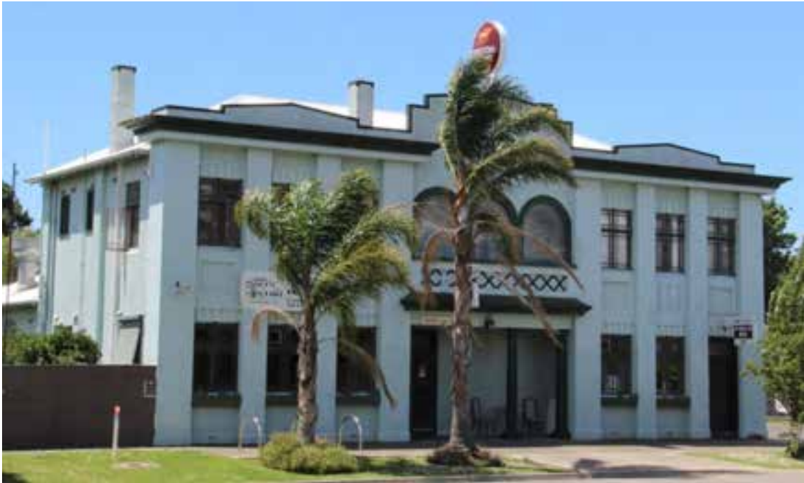
Figure D1. The two-storey symmetrical facade dominates the street with its Stripped Classical style. At the roofline is a low three-part parapet which sits above a bold cornice. Eight smooth-rendered engaged piers divide the facade into distinct vertical bays, with a large central bay with a recessed porch at ground level and balcony to the first floor.
