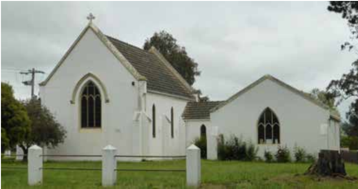
Figure D3. The east elevation of the church and its gabled-end fronts Lyons Street and is the main elevation viewed from this main street. The elevation comprises a large pointed-arch window with a label moulding. To the north of the church is a large hall constructed in a sympathetic style but is clearly a modern addition, with aluminium windows. A cement pier and metal pole fence runs along the south and east boundaries, with an interwar pedestrian gate at the south-east corner
