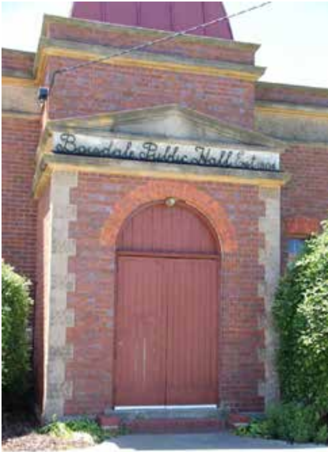
Figure D3. A detail of the original tuck pointed English bond entrance porch with its arched entrance, pediment, rendered dressings and metallic glazed bricks.
