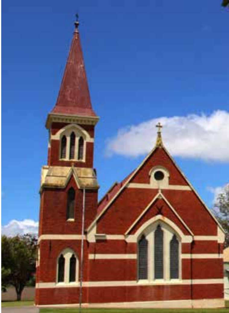
Figure D1. The church is constructed of handmade, tuck pointed red bricks, with a rendered plinth and gabled roof clad with corrugated iron. Four horizontal bands of decorative render (overpainted). run across the facade, creating dominant lines across the face-brick.
