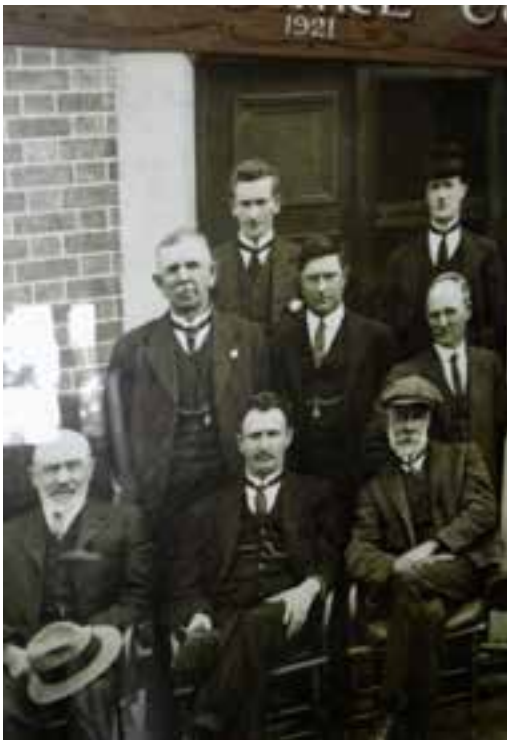
Figure H2. View showing the original finish of tuck pointed red brick walls, unpainted rendered architraves and timber doors, with Councillors in 1921 (RDHS).
