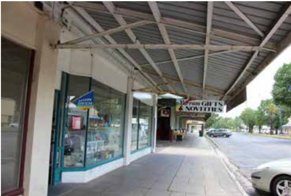
Figure D4. The shopfronts are covered by a wide cantilevered verandah with a skillion-roof (with modern cladding), which retains the original metal structure underneath. The shopfronts at ground level are early timber-framed windows with recessed entrances.
