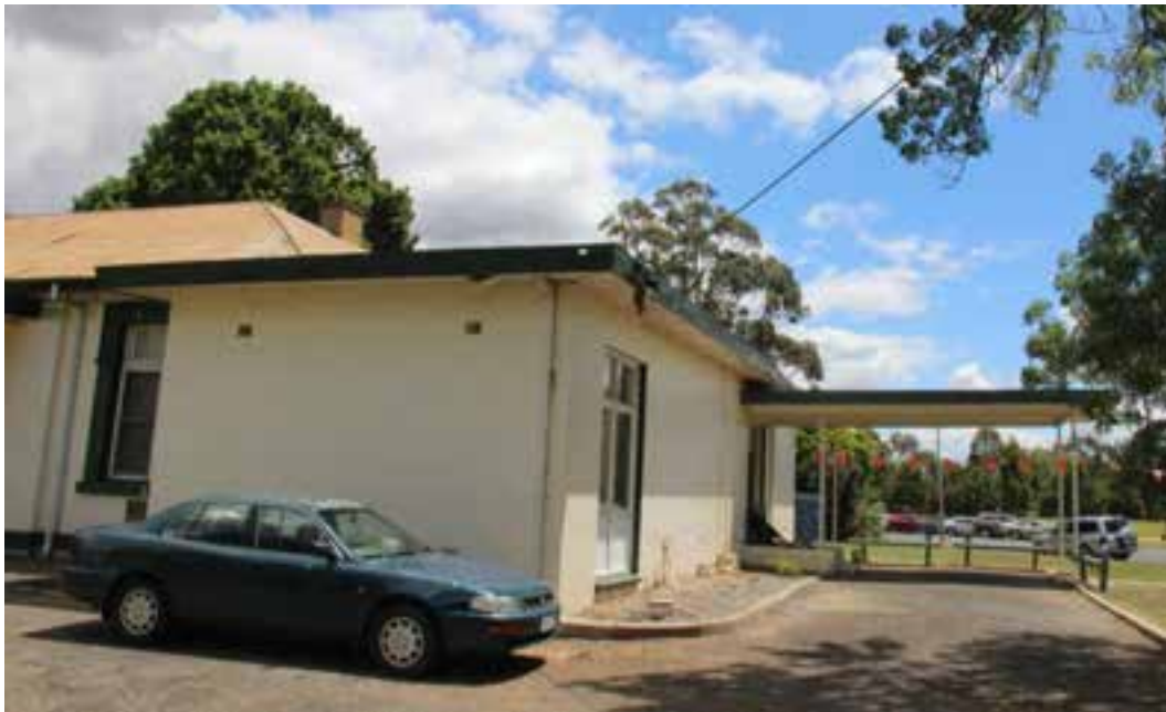
Figure D4. The large unsympathetic addition and carport was added to the north elevation in 1961, this is a cement-brick construction with a flat roof.
