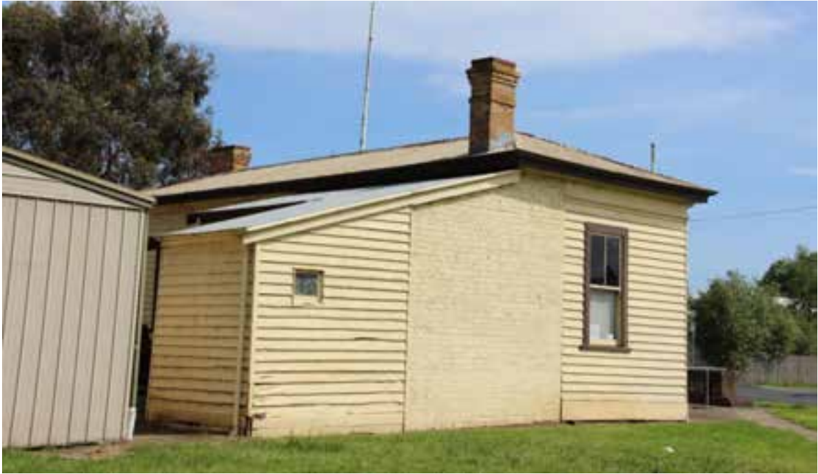
Figure D4. The south-east elevation, showing the two later additions with a skillion-profile roof. The brick section appears to form part of the chimney (reconstructed after its relocation in 1975).
