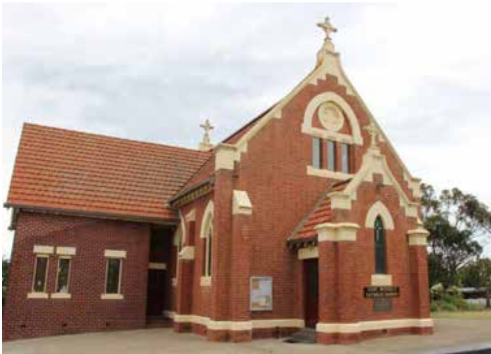
Figure D2. Projecting rafter ends are exposed beneath the eaves of the church. The two front bays of the side elevations of the 1916 church remain visible. Each bay has a pointed-arch window; set within is a trefoil above a pair of leadlight windows (with a diaper pattern and
