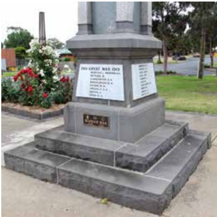
Figure D1. The bluestone quarry-faced stepped plinth, finely tooled pedestal, and the base and capitals of the cenotaph piers. Hand crafted marble plaques for WW1 and a new machine made bronze and paint plaque for the Korean War.
