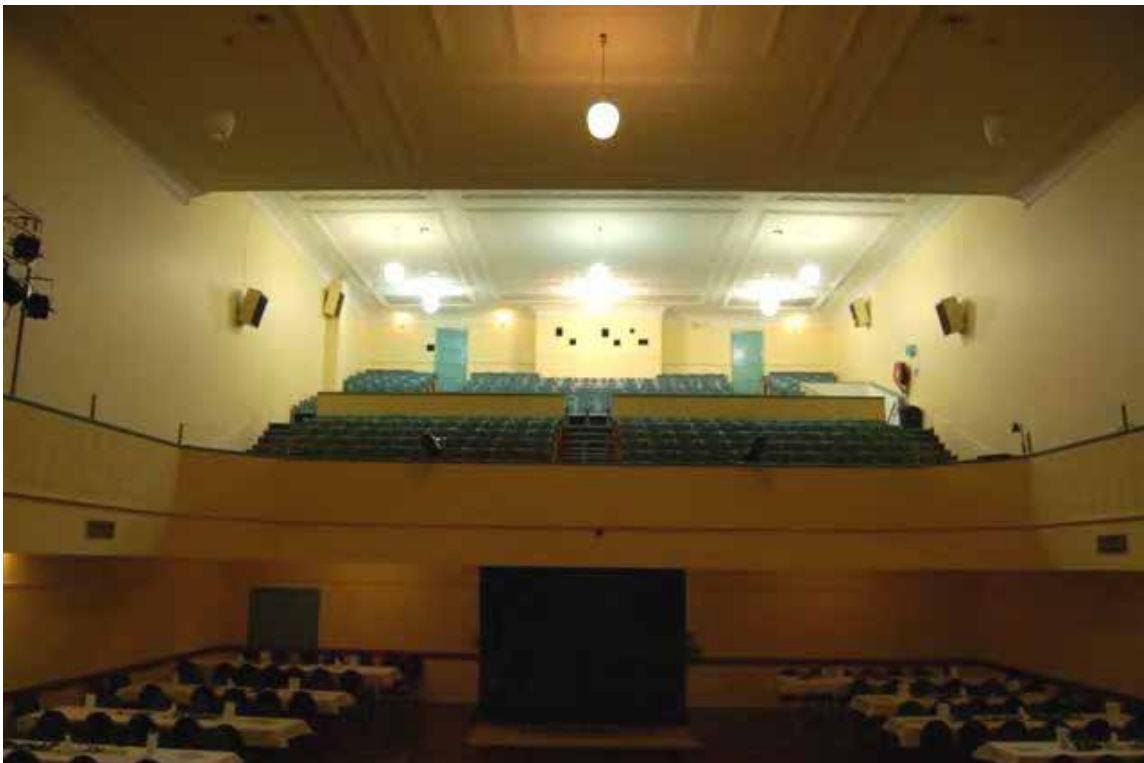
Figure D5. The auditorium also contains dress circle seating. Pressed metal clads the ceiling and the front of the circle and catwalks (Source: HV).
