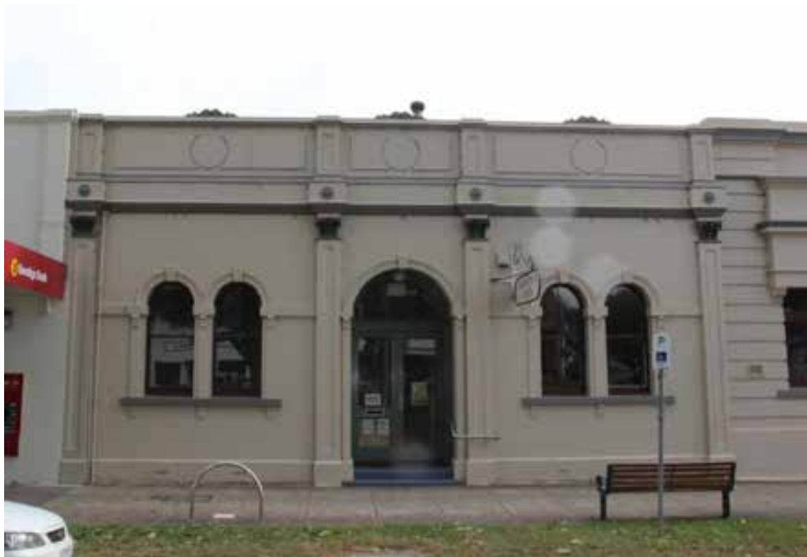
Figure D1. The facade of the Mechanics Institute (1886) with its smooth-rendered (overpainted) facade with Classical details and semi-circular arched openings.
