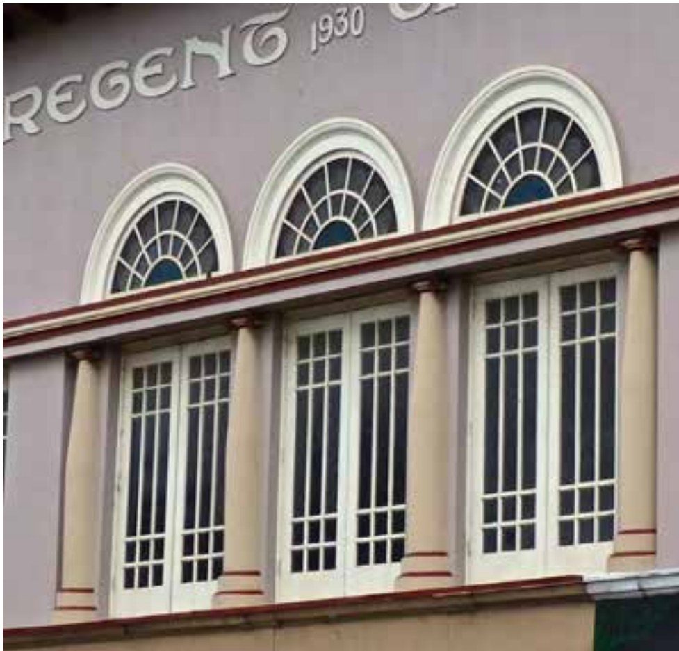
Figure D2. Detail showing the four Ionic columns with exaggerated entasis, separating the three pairs of French windows and supporting a moulded entablature with elaborate fanlights above.
