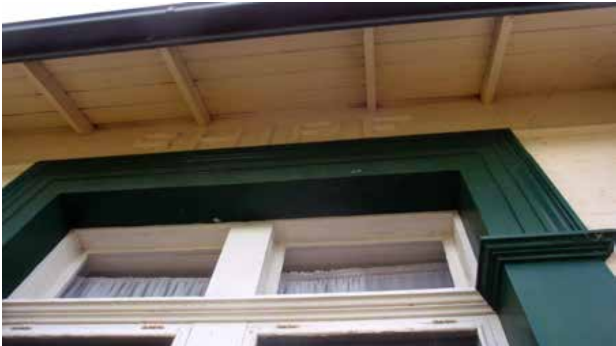
Figure D2. The words 'Shire Hall' and the date '1913' remain in raised letters beneath the 1961 eaves. The entrance and flanking windows are framed with original wide pilasters and sills (all overpainted in a heavy green colour). The eaves are from the 1961 changes, but the windows are original.
