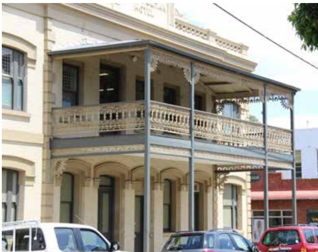
Figure D5. The many openings to the facade (except those under the verandah on the first floor) have bold segmental-arched mouldings to the top and are recessed within rendered surrounds. All windows have timber-framed one-over-one sash windows. The verandah posts are not original.
