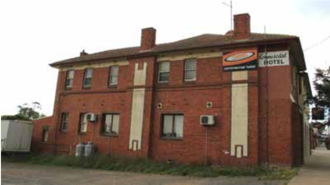
Figure D3. The south elevation has wide one-over-one sash windows. Two wide chimney stacks project from the elevation with a large vertical panel of decorative render in an ornate shape, framed in clinker bricks.
