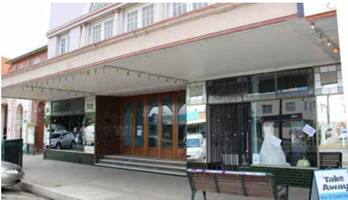
Figure D3. The cantilevered verandah covers the two elaborate shopfronts either side of the recessed entrance, reached by three marble steps.
