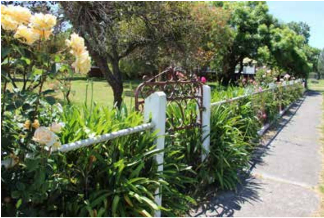
Figure D11. An interwar timber post, metal pole and chain wire fence runs along the front (east) boundary, with interwar decorative mild-steel vehicular and pedestrian gates at the entrance to the church and parish house.
