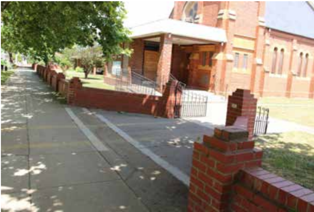
Figure D6. A red brick fence, with mild-steel gates lines the north, east and south boundaries of the property. The plaque on the right pier of the church entrance gates states that these gates were dedicated in 1950.
