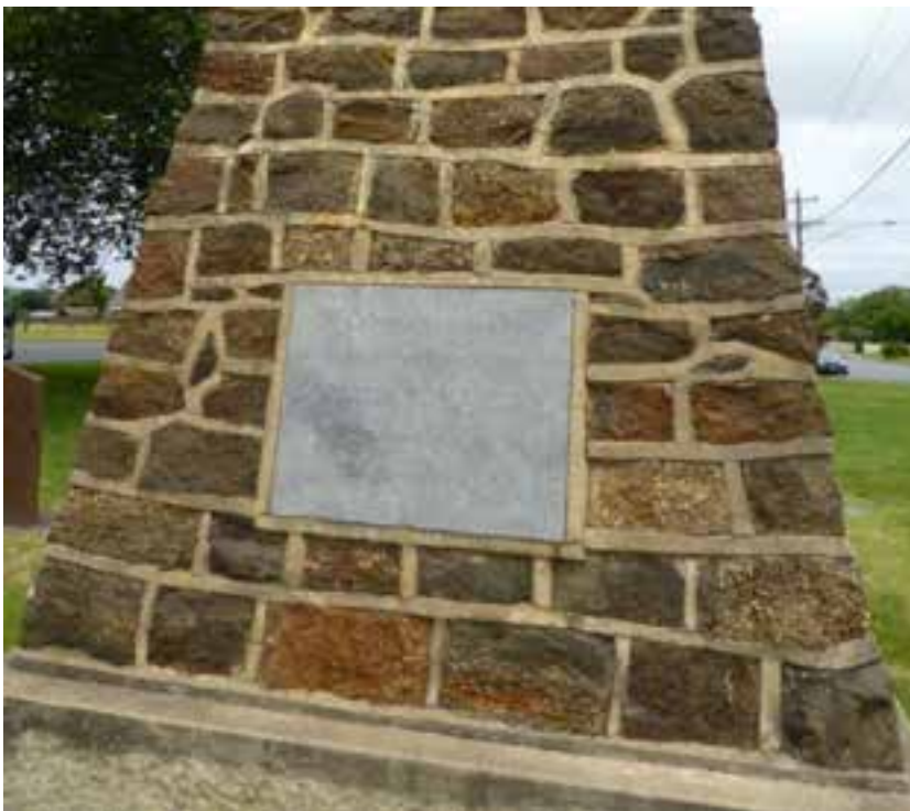
Figure D4. Detail of the 1927 Angus McMillan cairn, showing the local stone blocks, heavy protruding lime- mortar joints, 'concrete' plinth and marble plaque with hand cut incised lettering.
