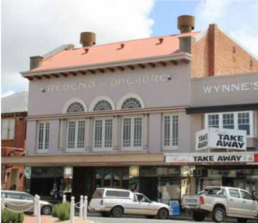
Figure D1. The theatre is a red-brick construction, visible on the side elevations where it extends into the gable ends, but concealed by decorative painted render on the front façade. The gable roof is clad in Colorbond deck, which replaced a former tile roof.
