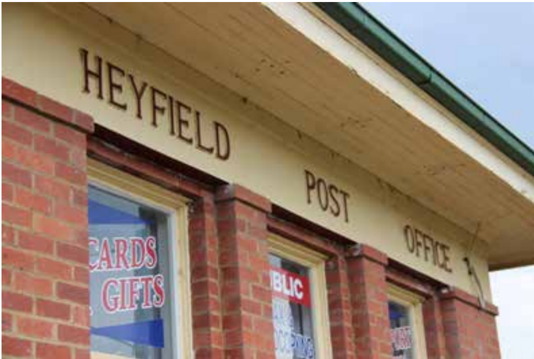
Figure D2. The wide eaves which are timber lined, and the name of the post office on the smooth band of decorative render.
