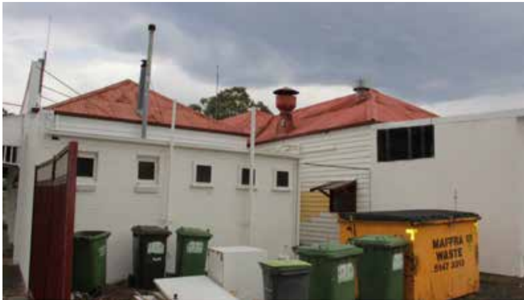
Figure D5. The rear (south) elevations, dating to the Victorian period, are clad in weatherboard, with the hipped roofs evident above.
