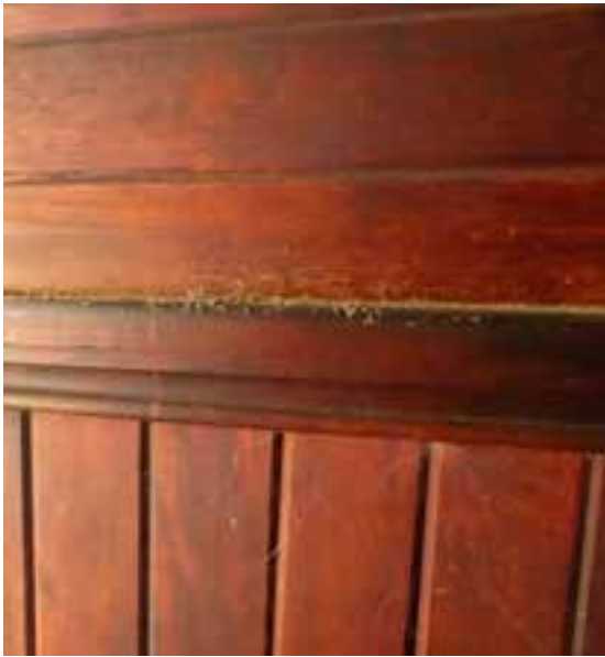
Figure D2b. Interior showing a detail of the carpentry of the red pine timber lined walls and dado.
