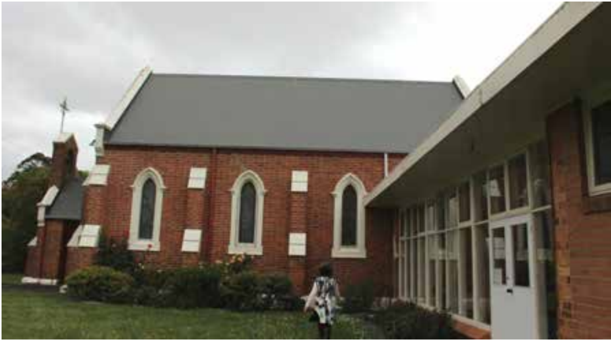
Figure D5. The east elevation. Three bays of the east elevation are visible. The c1960s cream brick addition adjoins the church in the fourth bay, at the rear of the church.
