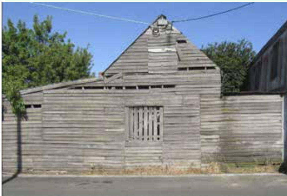
Figure D7. A timber outbuilding remains on the east boundary, which is an early stable (date not confirmed). It has a gabled roof with a filled in opening in the gable end, and another one below, and skillion additions off the long elevations.
