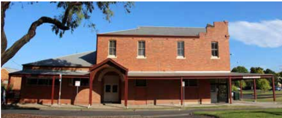
Figure D3. The parapet to the facade steps down on the side elevations, revealing the hipped roofline (with a gablette facing north), particularly from Foster Street. The first floor retains four original two-over-two sash windows with radiating voussoirs above and rendered sills.
