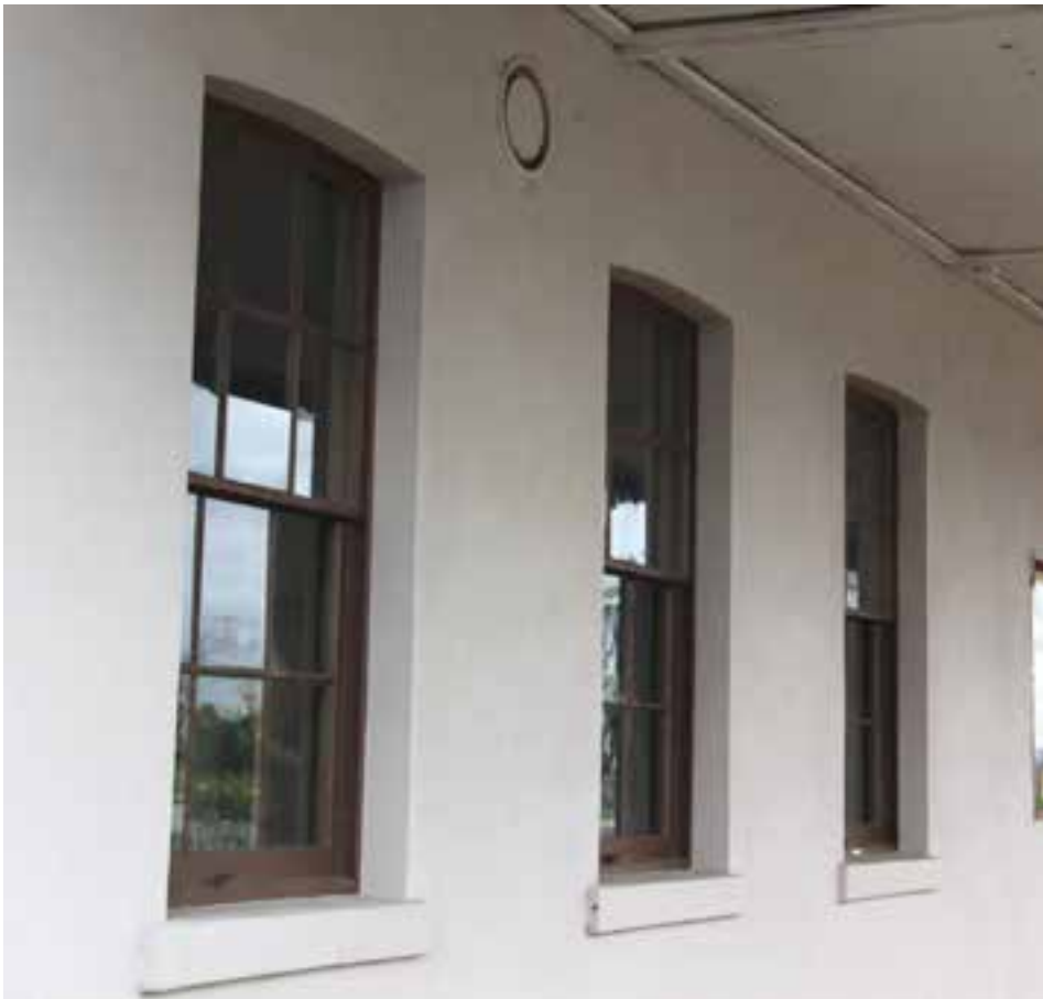
Figure D3. The ground level retains three original six-over-six sash windows on the southern elevation. All openings to the south elevation have radiating voussoirs above, and the windows have projecting sills (all rendered and overpainted).
