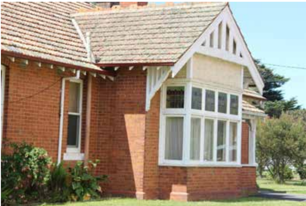
Figure D8. The gabled bay on the south elevation has a box window, with the top portion of the wall above the windows covered with rough-cast render, with a timber valence and large timber brackets to the gabled end.
