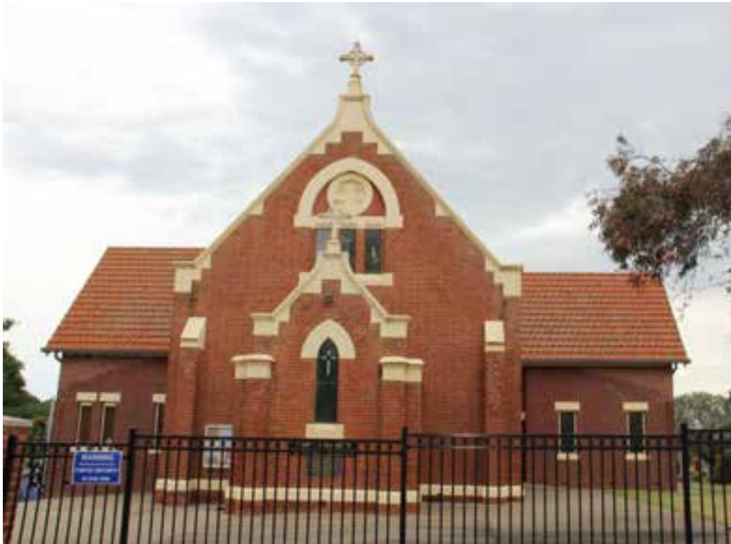
Figure D1. The tuckpointed red-brick church has a gabled roof clad with terracotta tiles, with rendered dressings and coping (overpainted) to the gable parapets, buttresses, plinth, and sills and lintels of the openings. Central to the façade is the gabled entrance porch, below the large pointed-arch window to the gabled end. Two substantial transepts were constructed (c1969 and c2000), projecting to the east and west.
