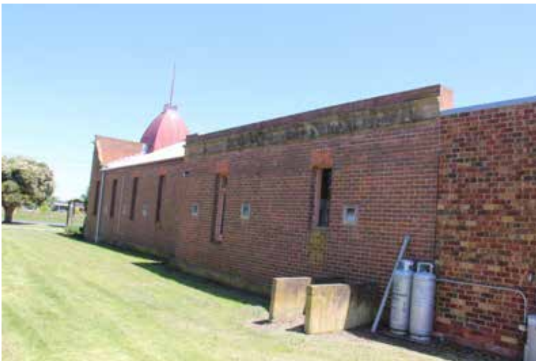
Figure D4. The south elevation showing the rear of the parapet which continues onto the side elevations. The windows have the same treatment as those on the facade. The rear section of the 1904 building has a parapet with a band of roughcast render.
