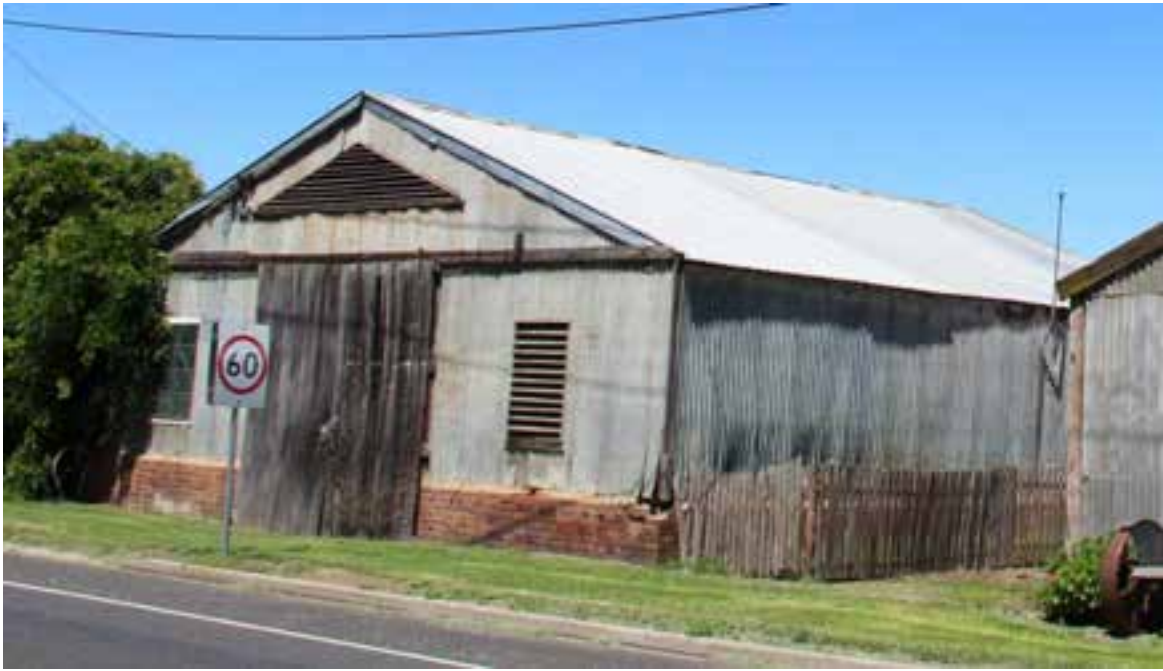
Figure D3. The blacksmiths and wheelwrights building at 37 Main Street. The gabled roof building retains its original sliding timber door, galvanised iron cladding and brick plinth and some timbered louvered openings.
