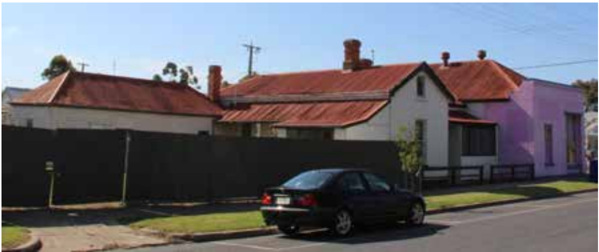
Figure D4. View showing the significant shop, residence and early large hipped-roof outbuilding. Off the south elevation of the house is a skillion-roof verandah clad in galvanised corrugated iron.
