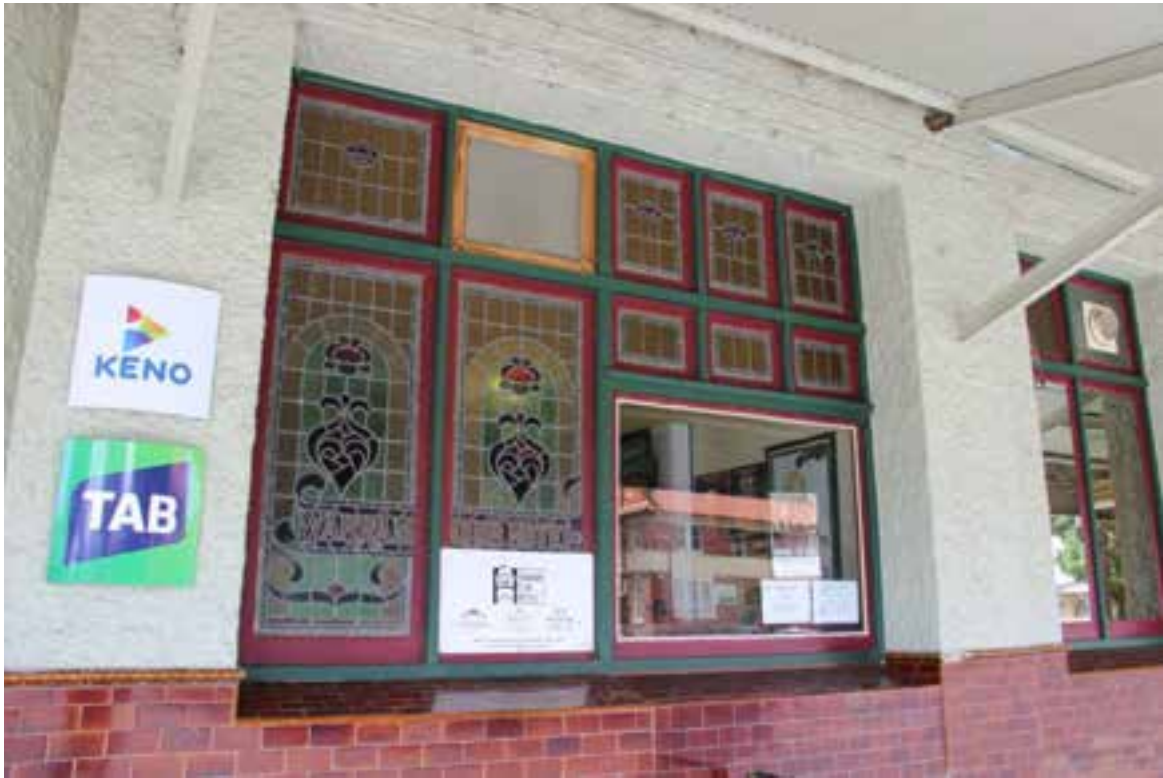
Figure D5. This photo shows the leadlight window group to the south (right) of the northern corner entrance. This is the only altered opening to the facade, as it originally had an entrance door in the right half (since closed over sympathetically). The leadlight to this window contains the words 'YARRAM CLUB HOTEL'.
