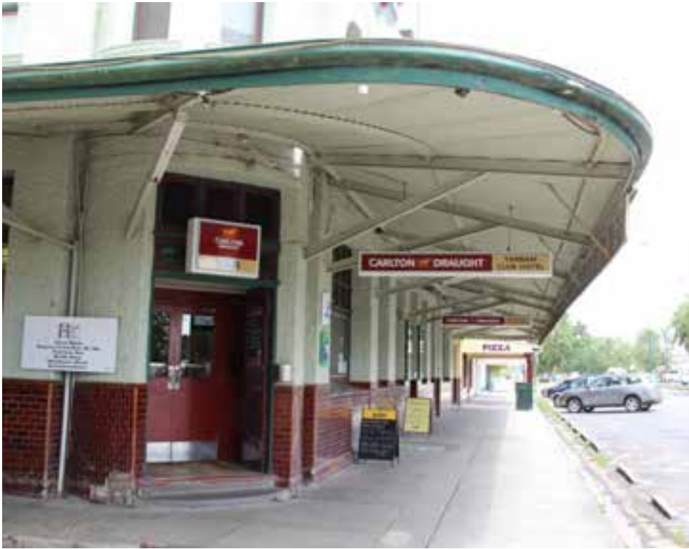
Figure D3. The wide cantilevered verandah runs across the facade and returns on part of the north elevation, with large rounded corners. It has corrugated iron cladding (overpainted) to the roof and retains the original metal support structure underneath. The ground floor has glazed brown tiles to the dado level with roughcast render to the top 2/3 of the wall (overpainted).
