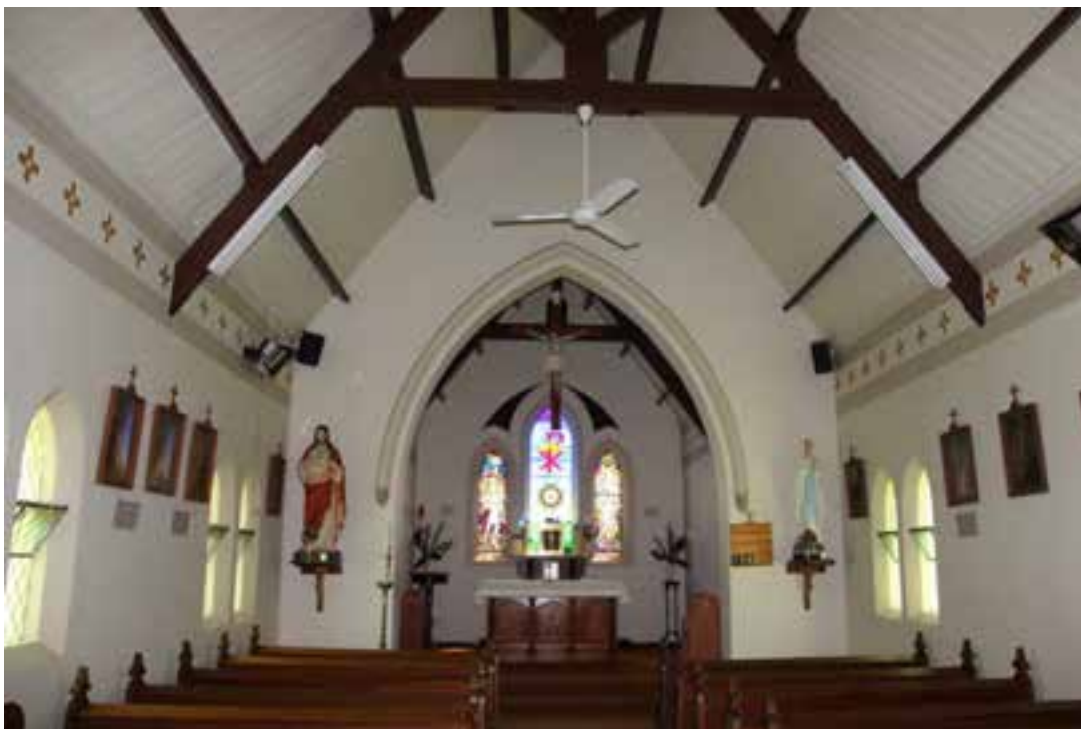
Figure D4. The interior of the church has a timber-lined ceiling, with exposed timber trusses. The walls are rendered, with ruled incised lines to create an ashlar effect. The nave is separated from the chancel by a pointed-arch entrance with a decorative label moulding.
