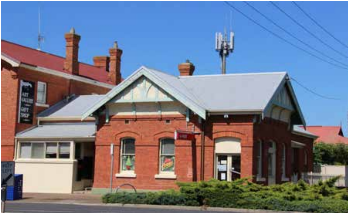
Figure D5. The main elevations of the post office, and the verandah to the left (with later in-fill). The two jettied gabled-ends have roughcast render and timber strapping, creating a half-timbering effect. Note the historic picturesque skyline of roofs and chimneys.
