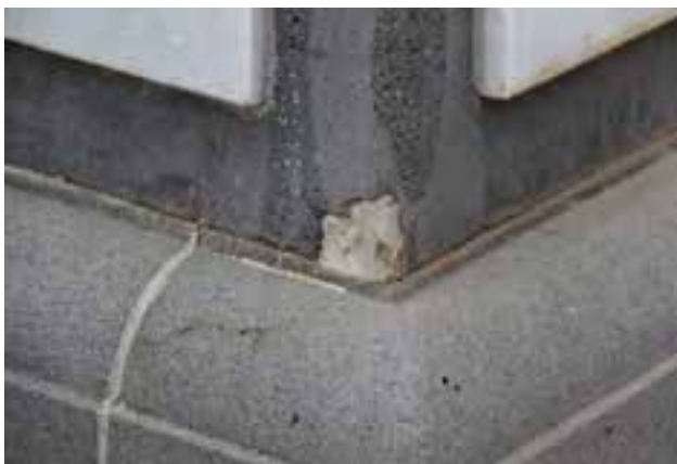
Figure D2. Detail of damaging repairs using a 'plastic type' substance in the joins instead of
