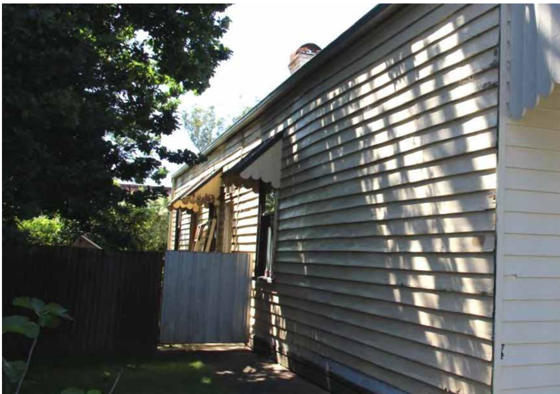
Figure D2. The north elevation has openings to the rear of the building, including three with skillion-roof hoods and round-edged cladding to the sides, like the verandah. One has since been rectified by owner, due to severe rot (Feedback from owner 9 May 2016).
