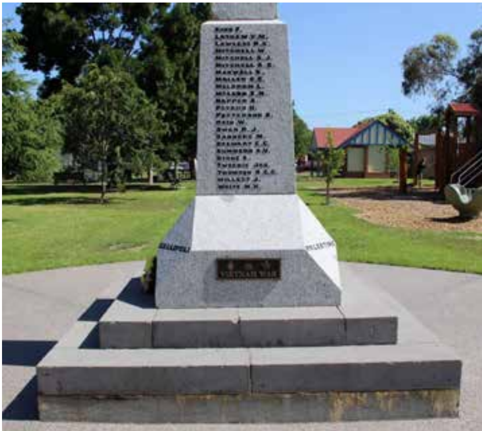
Figure D3. Detail of the concrete foundations, bluestone steps, names ( eg GALLIPOLI) incised into the granite, and names on soldiers in lead. Modern bronze and painted plaque.
