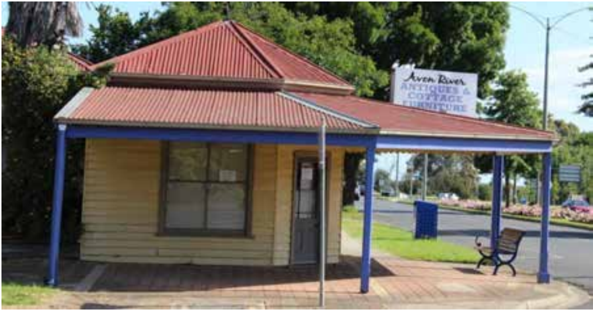
Figure D3. The small weatherboard corner shop has a faceted hipped roof clad in galvanised corrugated iron (painted). The original wide verandah extends over the pedestrian footpath, is clad with galvanised corrugated iron, has round-edged palings to the sides, and is supported by shop-chamfered timber posts, some with a timber base.
