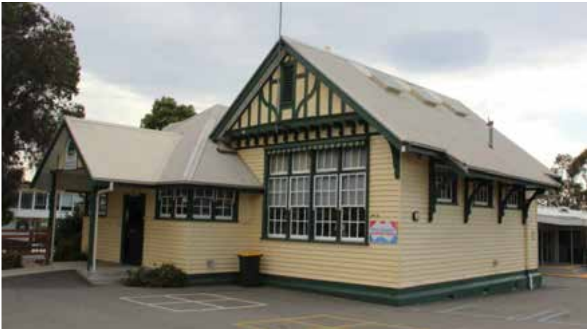
Figure D6. The front (east) elevation faces Temple Street. The weatherboard building has an asymmetrical plan and a complex hip-and-gabled roof recently clad with Colourbond. The wide timber-lined eaves are supported by large ornate timber brackets. The multiple gabled ends have a flying gable with roughcast render and timber strapping (with curvilinear details) to the gabled
