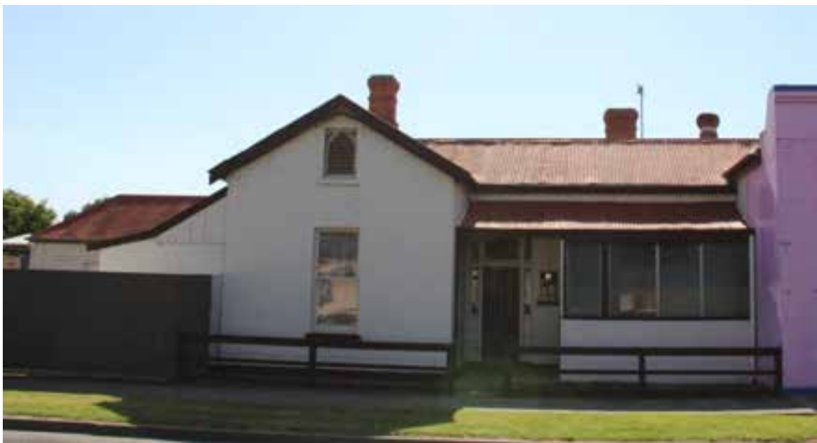
Figure D2. The residence is attached to the south of the shop, fronting Tyers Street. The brick (overpainted) residence has an M-hip roof, and a projecting gabled-bay to the facade, all clad in galvanised corrugated iron (overpainted). The facade has a projecting gabled-bay to the left and a slightly-concave verandah fills the recessed portion of the facade to the right.
