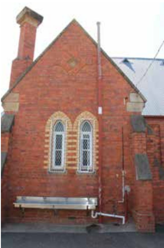
Figure D4. At the rear of the west elevation is a vestry (1893) with a parapeted gable, large chimney (the top half angled) with a wide rendered cap. The west side of the vestry has an
