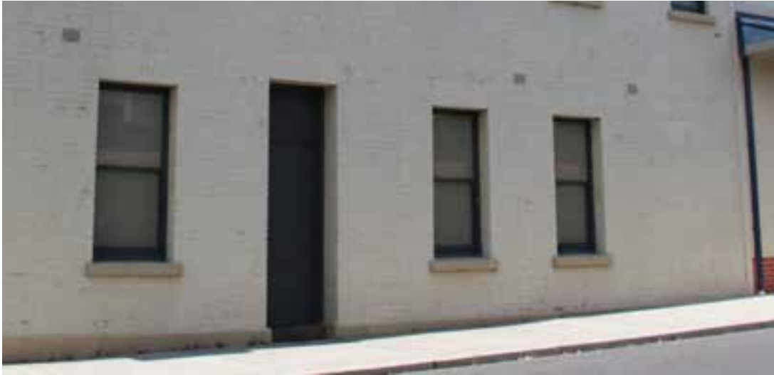
Figure D3. The west elevation fronting Purdy Lane retains the original openings (one at the south end has been closed over). The square-headed openings have radiating voussoirs and a rendered sill.
