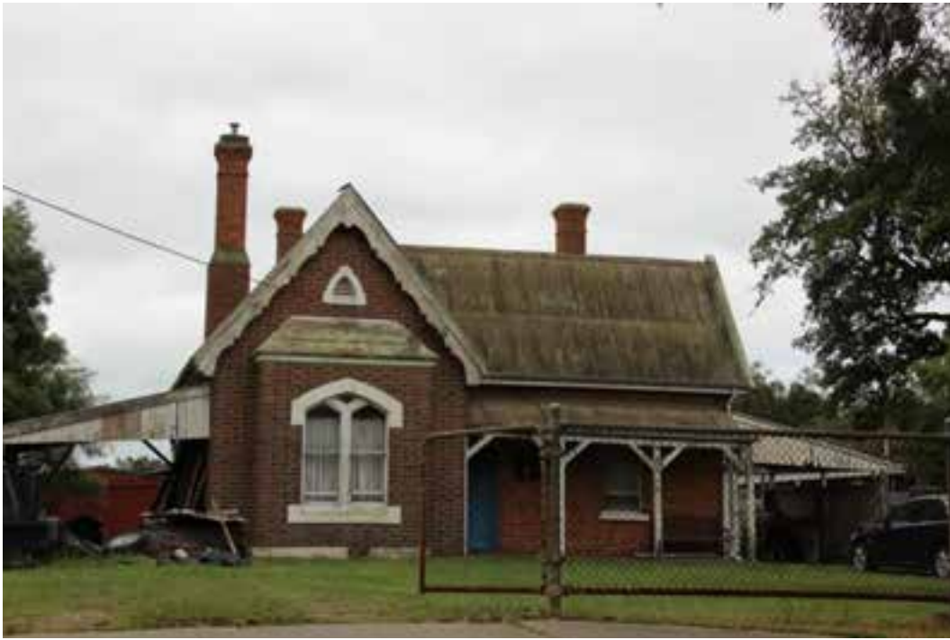
Figure D1. The brick manse has steeply-pitched gabled roofs, clad with lapped corrugated iron. From the street view, it is evident that the recessed portion of the house is constructed of red brick, while the projecting gabled-bay to the left of the facade is constructed of brown brick (this bay probably built in 1891).
