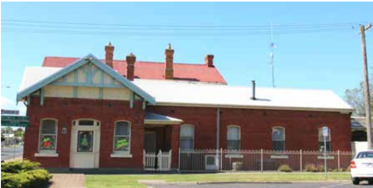
Figure D6. The south elevation of the post office and residence to the rear. The entrance at the centre of the gabled-bay has been altered to become a window. A section of the early (possibly original) fence remains beneath the porch. Note the historic picturesque skyline of roofs and chimneys.
