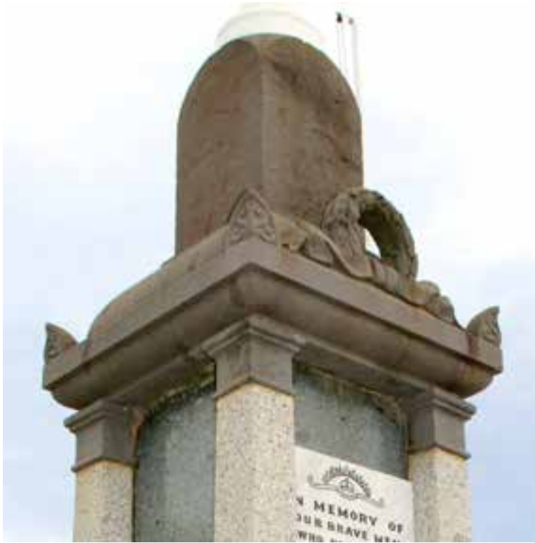
Figure D3. Detail of the top of the cenotaph showing finely tooled bluestone, polished Harcourt granite piers and Orbost granite panels, with some water damage occurring at the top of the panels.
