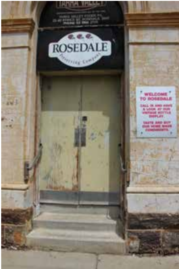
Figure D5. A detail of the facade and entrance showing the unpainted original local stone plinth ruled lines to the unpainted rendered wall planes, and the later doors, metal balustrades and concrete steps.
