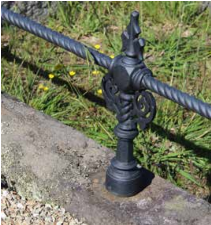
Figure D4. Detail showing lichen on the bluestone plinth, and 'restored' cast iron rail and post.
