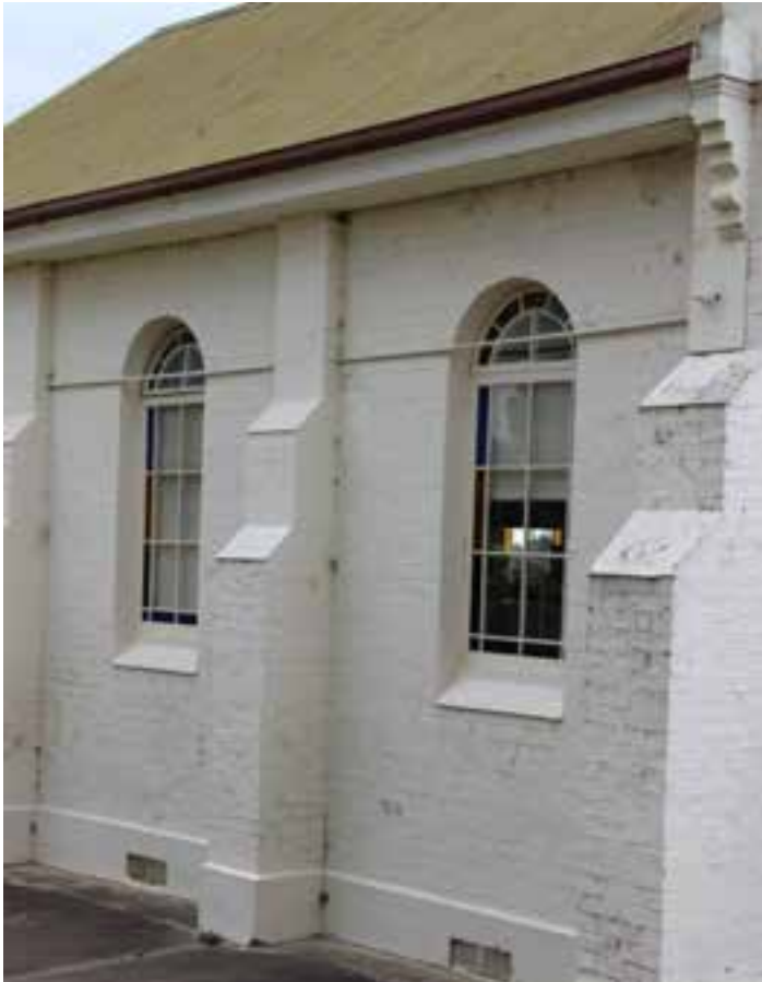
Figure D4. A detail of the semi-circular arched windows shows that they are multipane windows with a border of blue and red-coloured glass. The round segmented section at the top may be an
