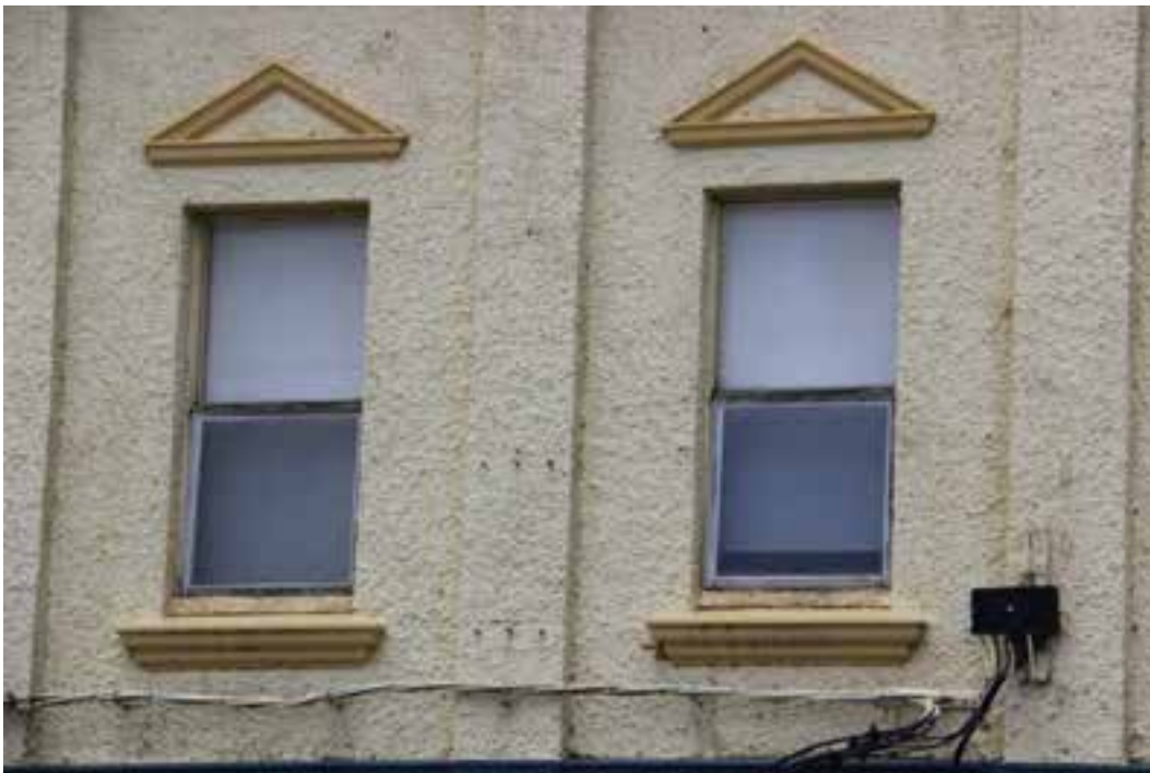
Figure D2. A single window appears in each bay (formed by the pilasters) to the first floor. The windows are one-over-one timber sashes with a moulded sill and moulding above that forms an abstracted Classical pediment.
