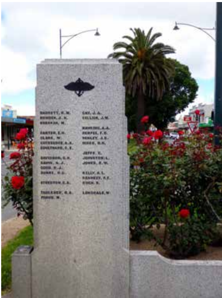
Figure D3. Illustrates the design of the WW2 monument, good condition of the polished granite, and black painted hand cut, lead lettering.
