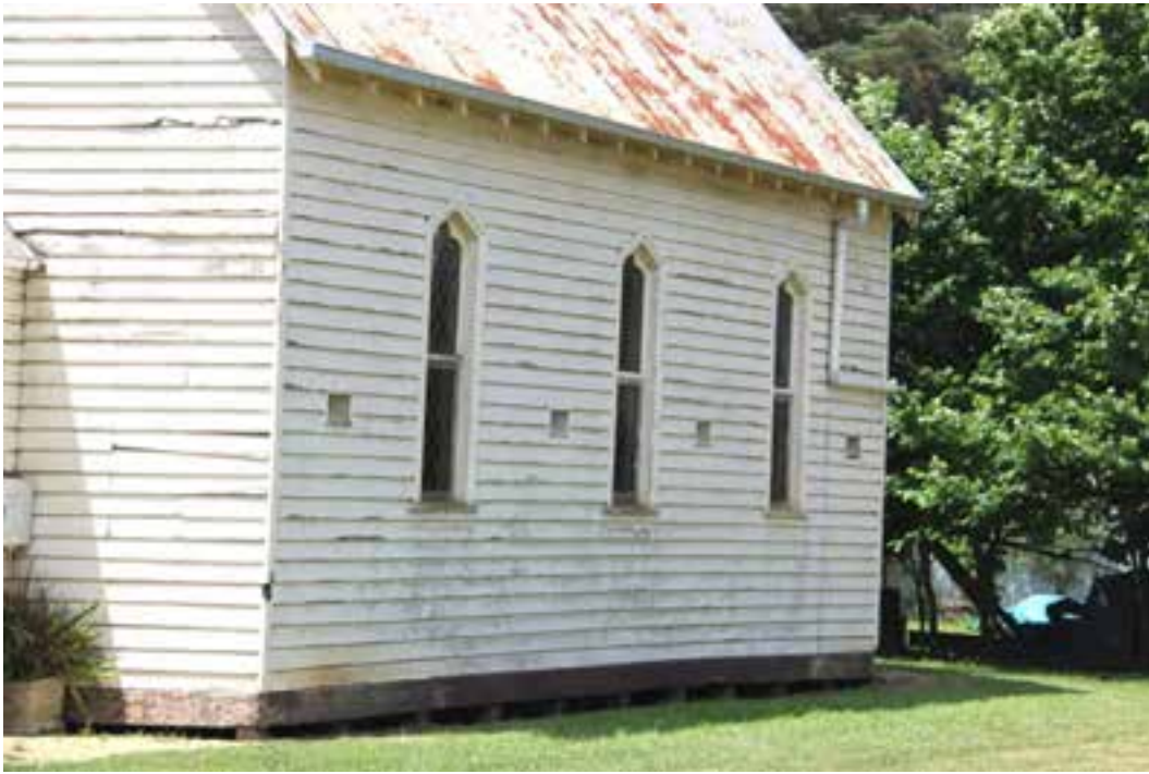
Figure D2. The south elevation with the three leadlight windows in a diaper pattern and trefoil motif to the top, set within the pointed-arched timber frame.
