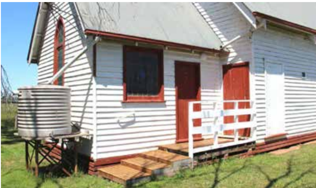
Figure D4. The north elevation comprising the square leadlight window to the chancel. Two timber doors provide access to the chancel and nave, while the third appears to not be in use.
