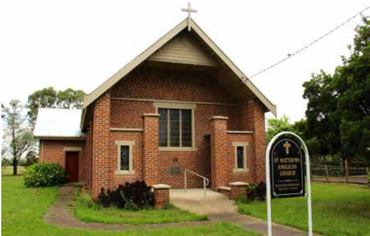
Figure D1. The church is constructed of handmade brown bricks and deliberately contrasting light coloured lime mortar, struck flush with the face of the brick, with a brick plinth and gabled roof clad in lapped corrugated iron (recently painted an appropriate colour). The roof projects forward at the façade, creating a deeply recessed entrance porch for the symmetrical façade.
