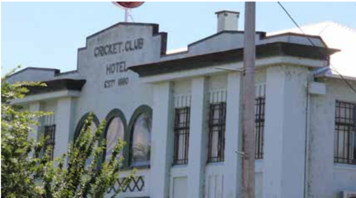
Figure D2. The central parapet to the facade reads 'CRICKET CLUB HOTEL ESTD 1880' in relief. Below are three round-arched openings, with rendered frames, which open into the balcony to the first floor. The windows are ornate steel-framed multi-paned casement windows, with opaque glass to the outside panes.
