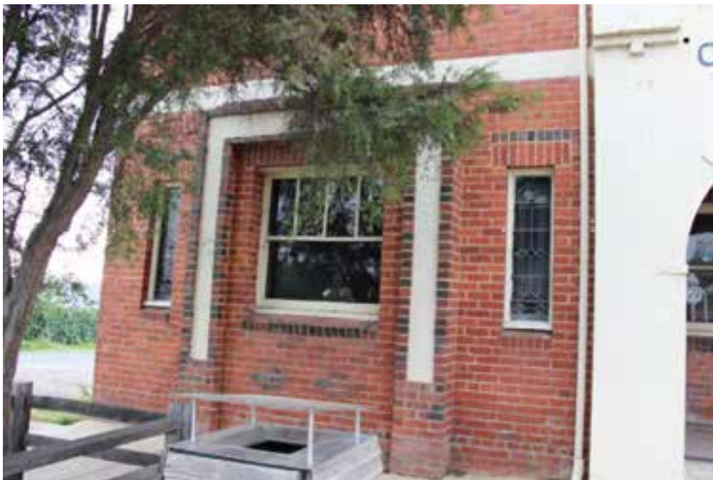
Figure D2. The openings to the building generally have a row of soldier (dark-coloured) clinker
