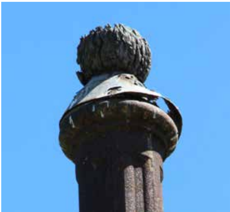
Figure D3. Detail of the fluted metal column, capital and 'flaming' metal orb.
