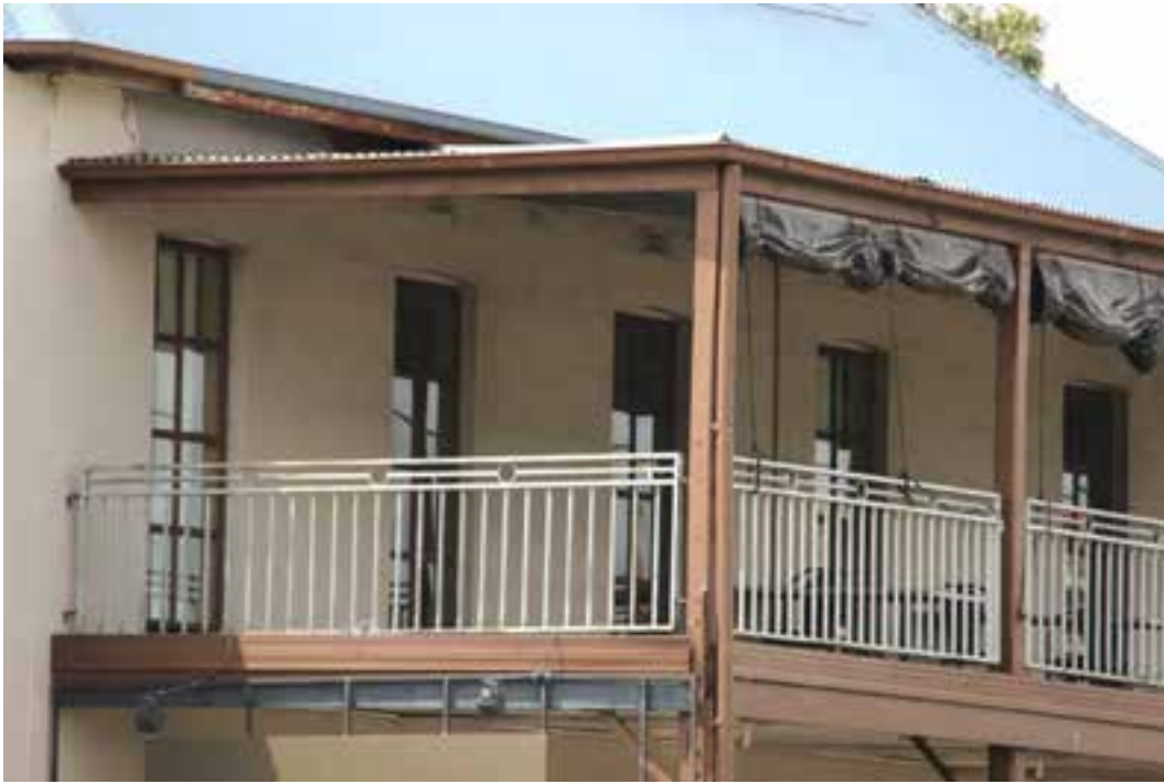
Figure D2. The tall openings to the first floor of the south elevation are all original (with modern multi-paned windows that replaced the original French doors).
