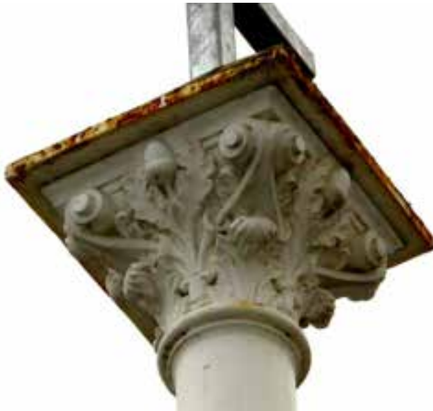
Figure D4. Detail of white painted rusting cast iron column with recent metal cross above.
