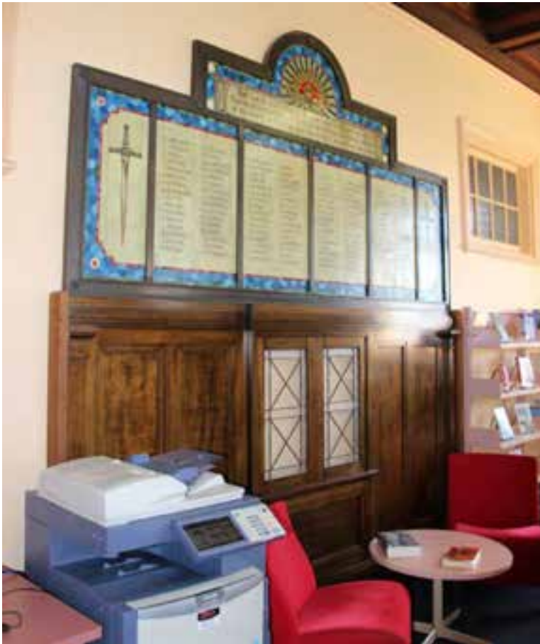
Figure D6. The World War I Shire honour roll, that forms one part of the opus sectile memorial held in the RSL club rooms of the 1922 Great War Peace Memorial Hall. Positioned below is timber panelling with a pair of leadlight casement windows, which originally formed a ticket box in the entrance hall, facing the entrance doors, above which the honour roll was erected.
