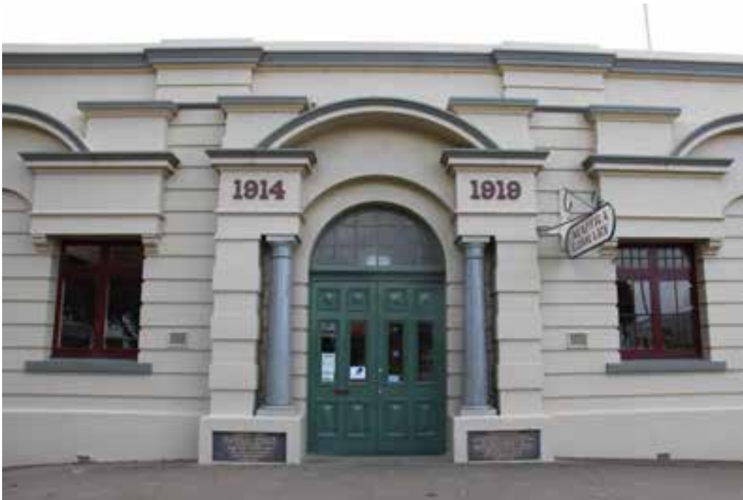
Figure D3. The elaborate entrance with the foundation and memorial stones and pair of polished granite columns with Tuscan capitals, which support the entablature which bear the dates '1914' and '1919'.
