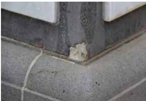
Figure D2. Detail of damaging repairs using a 'plastic type' substance in the joins instead of
