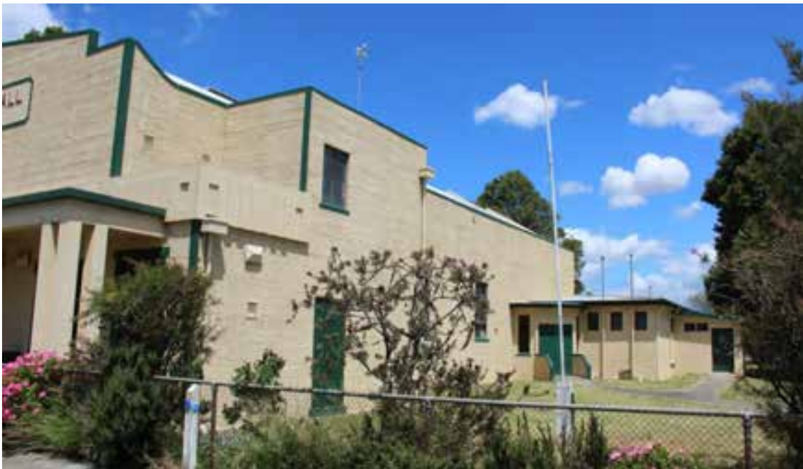
Figure D4. The west elevation has a timber ledged and framed door at the north end and 4 and 8-paned metal-framed windows with rendered sills. A large single-storey addition is constructed off the rear (south) and west elevation of the hall, which serves as the toilets.
