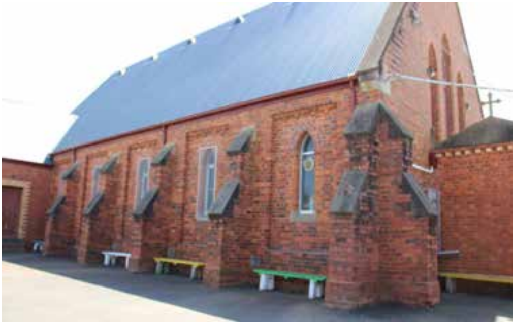
Figure D3. The west elevation. The pointed-arch windows of the side elevations have three rows of radiating brick voussoirs, chamfered bricks to the sides, and a renders sill. All of the windows have been replaced with modern aluminium-framed windows in a sympathetic style, most covered with a modern security grill to protect the windows in the sports grounds that surround the church.
