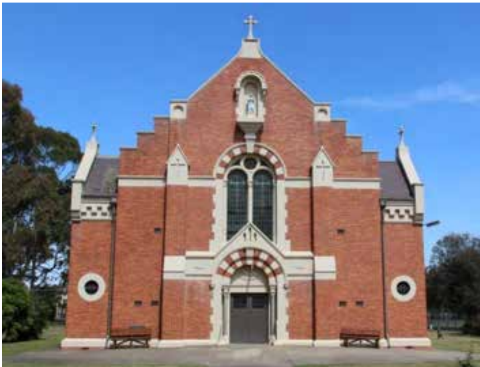
Figure D10. The 1924 church is a substantial red brick church with a (partly) rendered plinth and gabled roof clad in Welsh slate. Dominant features of the facade are the semi-circular arched
