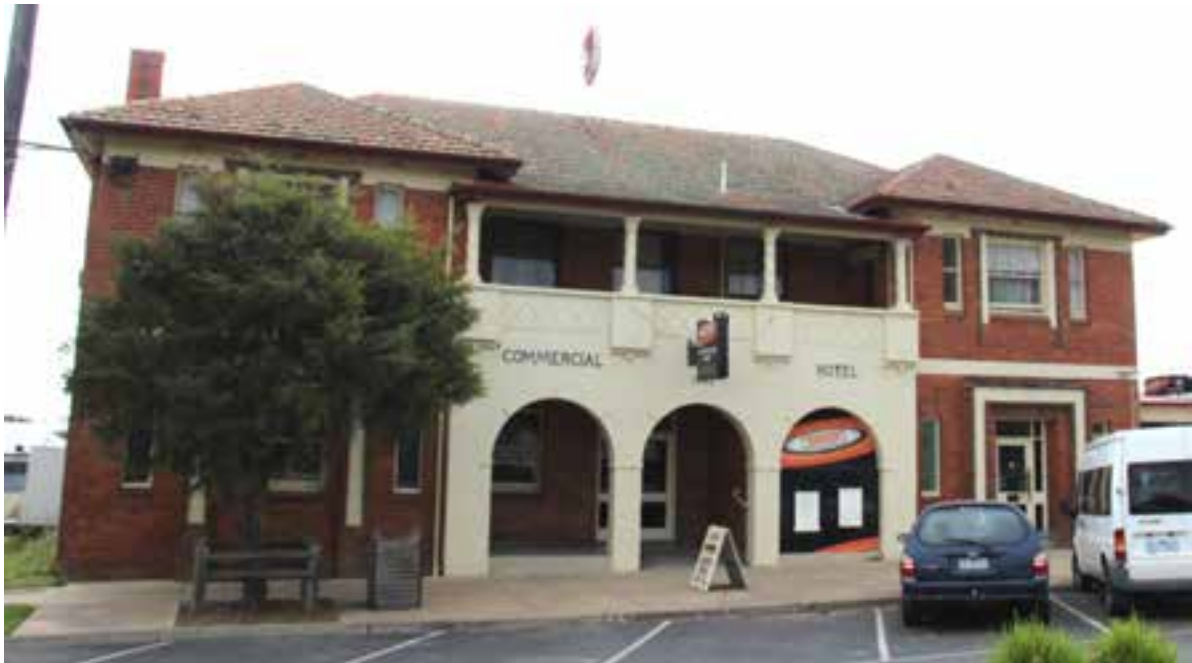
Figure D1. The two-storey red-brick building has a hipped roof clad with terracotta tiles with timber-lined eaves. The symmetrical facade has a two-storey hipped-roof bay at either end and a central rendered (overpainted) entrance porch (in the recessed section of the facade) which extends to the first floor to form a balustrade for a balcony.
