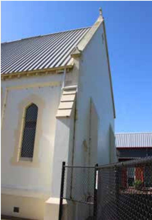
Figure D5. The rear (east) elevation has a simple treatment. It has a niche in the shape of a cross at the top of the gabled-end, like the facade, and two simple buttresses.
