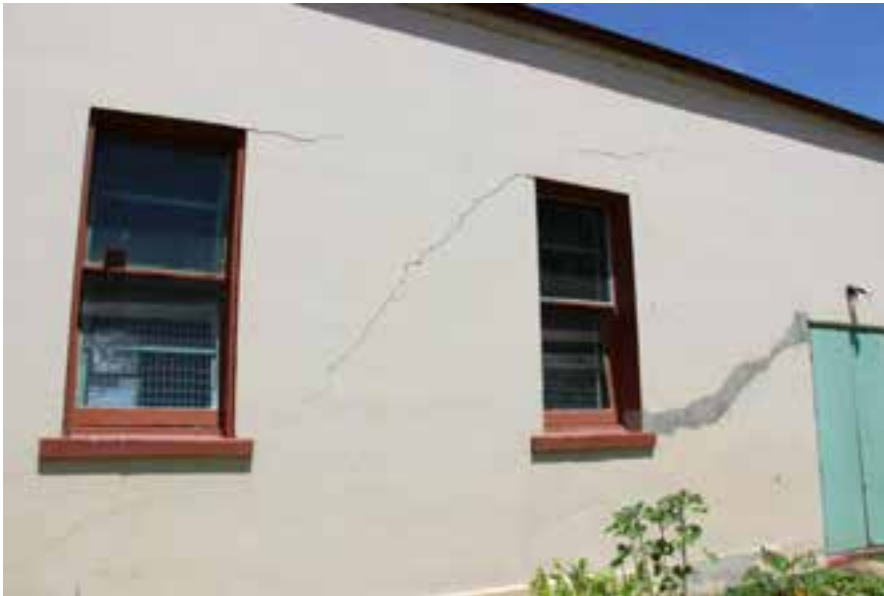
Figure D4. A detail of the windows on the north-east elevation, which are (later) timber windows. Note the cement repairs of a large crack.
