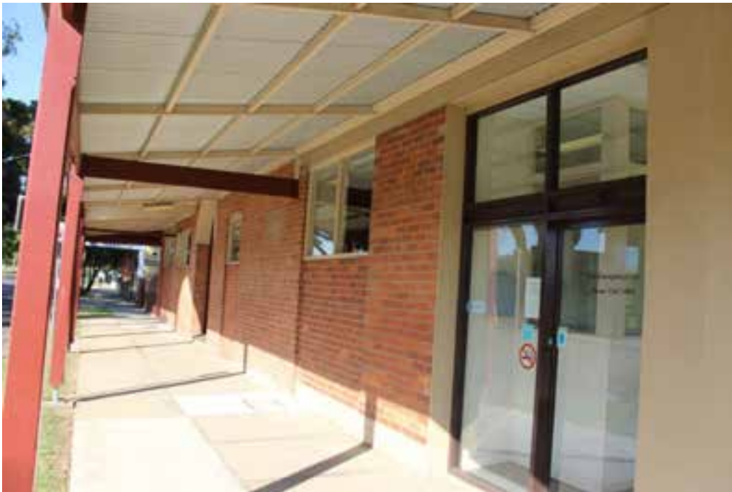
Figure D5. The ground floor on the west elevation retains part of the original external wall. Modern windows and doors have been inserted (in 1975). Small high-set windows have been inserted, in some cases in original openings (with the remainder of the opening bricked up).
