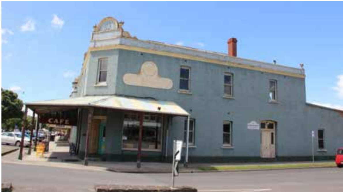
Figure D1. The two-storey building has a hipped roof clad with corrugated iron, and is constructed of handmade tuck pointed red-bricks (overpainted), with a brick plinth. Both main elevations have a rendered (overpainted) parapet above a bold cornice moulding; the southern elevation retains the urn at the end.
