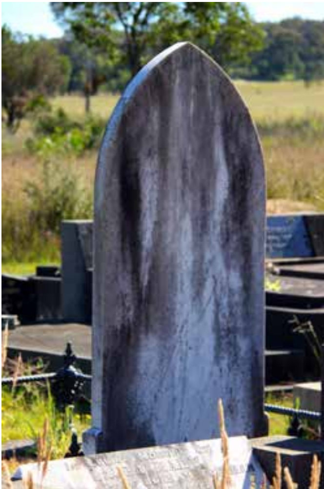
Figure D3. Back of the gothic memorial headstone showing black algae growth.
