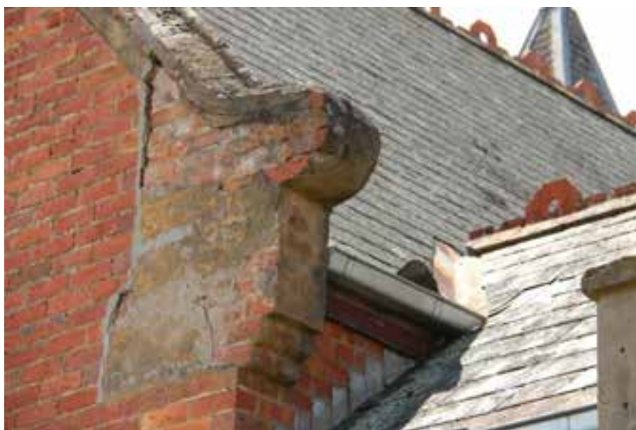
Figure D7. A detail of the cracking of the parapet coping in the rear gable-end.
