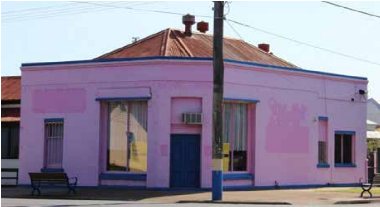
Figure D1. The large shop has a hipped roof clad with galvanised corrugated iron (overpainted) and a number of recent round metal vents to the roof. The shop is constructed of handmade red-brick (all overpainted) with a small brick plinth. The main elevations of the brick shop front Tyers and Blackburn Street, with a chamfered corner entrance and rendered parapet.
