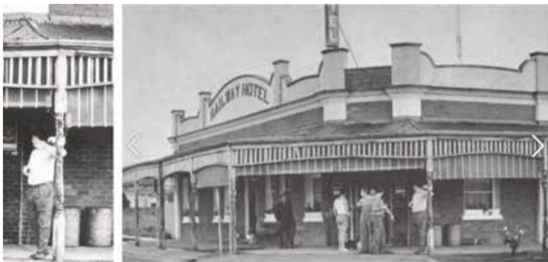
Figure H4. Photo showing the unpainted red brickwork, and the window and door fenestration which appears to match the Victorian era windows shown in Figures H1 and H2. The highly decorative turned timber posts and timber verandah valance are typical of the Federation era design ( see inset detail). Although this photo was taken in 1975 the building, including the verandah, as seen in this photo, is virtually unchanged from its appearance when it was built c1918.
