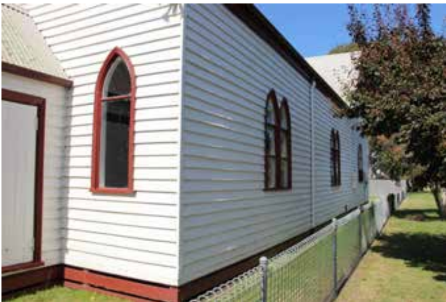
Figure D5. The south elevation of the hall has three pairs of pointed-arch windows (with clear glass) with central hoppers. There is excellent underfloor ventilation between the gaps in the base boards.
