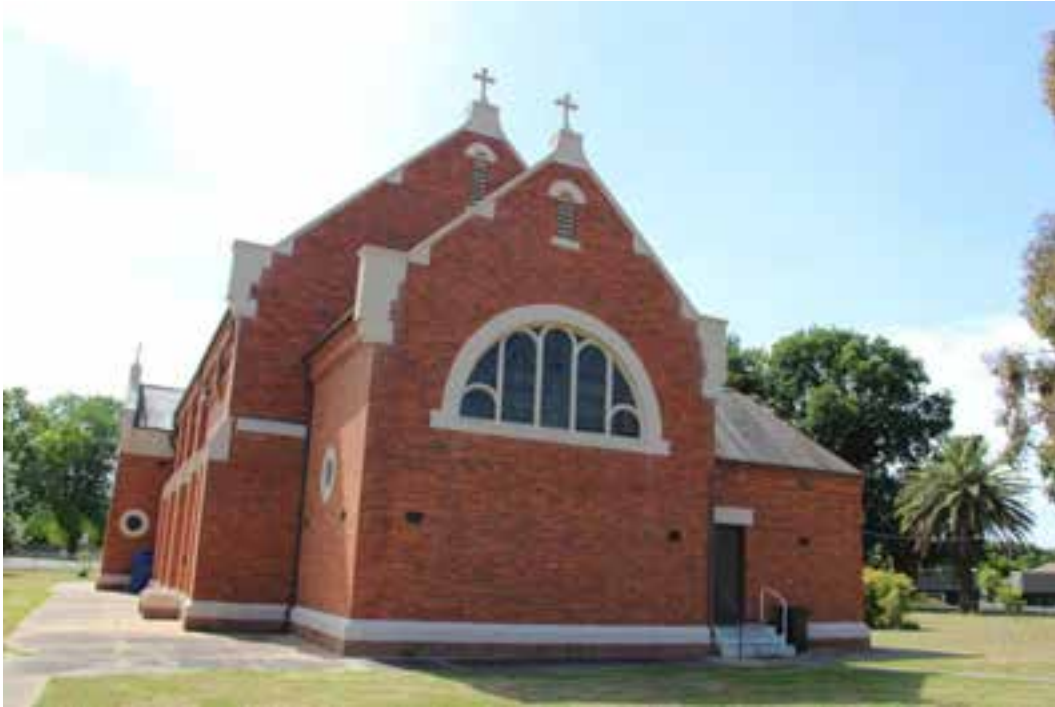
Figure D13. The west (rear) end of the church has a large chancel with a parapeted gable that imitates the details of the elevation behind. Its west face has a large high-set Diocletian window with a five-part window with leadlight. A small hipped-roof vestry projects off the south elevation of the chancel with an entrance off the west side and square-headed windows to the south side (Figure D12).
