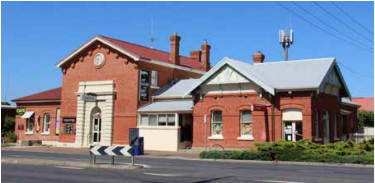
Figure D1. The main elevations of the (left to right) council chambers, two-storey court house and post office with the attached residence to the rear. Stylistically, the buildings are tied together by corbelled courses of brickwork that run horizontally below the eaves and at the tops of the windows, extending over the voussoirs of each window.
