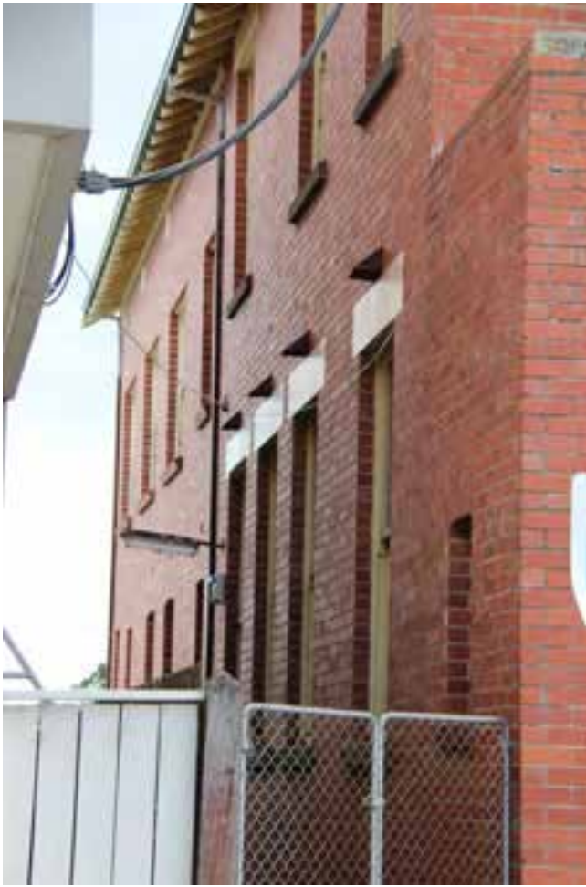
Figure D4. The south elevation. The 1950s addition to the first floor was built with wide eaves with exposed rafter ends, like the original 1913 section.
