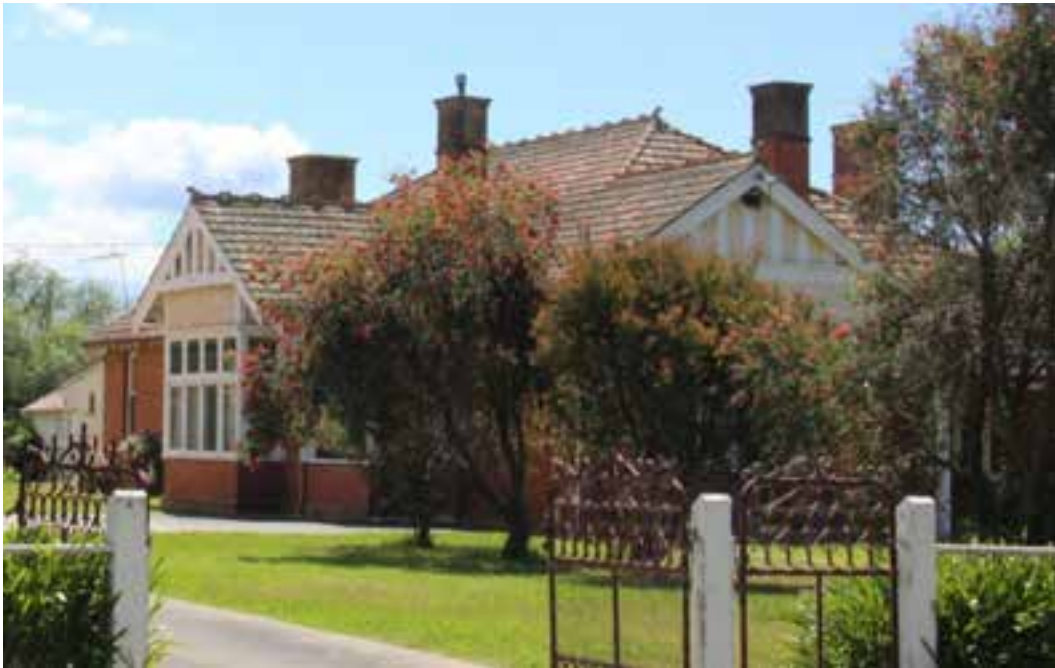
Figure D7. To the north of the church is the parish house (1904). The large red-brick (tuckpointed) house has a brick plinth and complex hip-and-gabled roof clad with Marseille terracotta tiles and terracotta ridge decoration.
