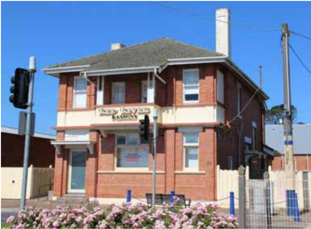
Figure D1. The facade (east elevation) with its low-pitched hipped roof, continuing over the projecting balcony to the first floor.
