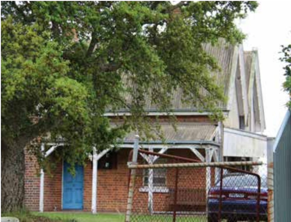
Figure D3. The two transverse gabled-ends of the east elevation have decorative bargeboards and what appears to be a render or plain cladding to the gabled-ends (previously face brickwork see Fig H1).
