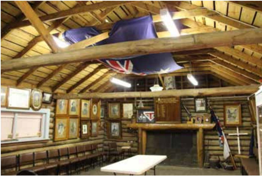
Figure D5. The interior of the log cabin is in very good condition and has a very high level of integrity, retaining its original timber elements. The interior walls are not lined, with the Yellow Stringybark logs evident.
