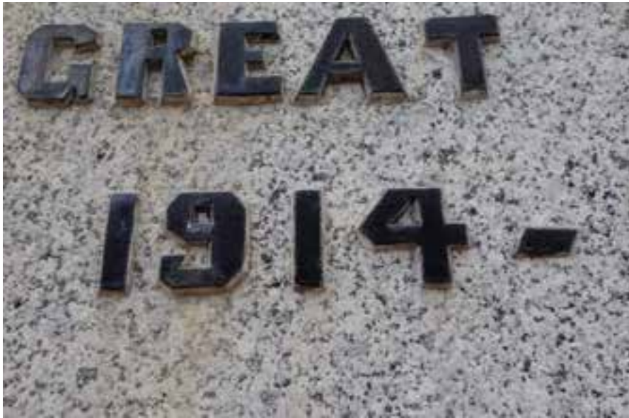
Figure D4. Detail of the polished granite surface, and hand cut black painted lead lettering, all in excellent condition.
