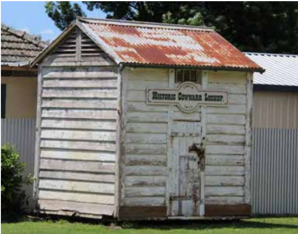
Figure D3. The small iron cage lockup with its gabled roof, half-round spouting and weatherboard wall cladding. It retains timber vents at the gable ends, a metal grill above the door, and its original (or an early) door with full-width hinges and a number of early locks.
