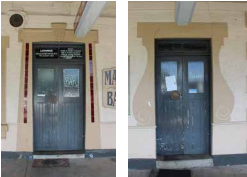
Figure D4. The surrounds to the doors of the facade are varied and elaborate. The main entrance has an Egyptian styled entrance comprising a rendered lintel, a bold keystone with vermiculation and tapered sides with a vertical line of red glazed tiles. Other entrances have a surround with a rendered lintel which extends to the sides in large lobed patten at the base.
