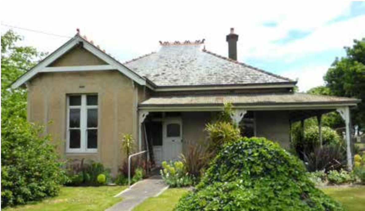
Figure D1. The 1914 concrete house fronts Lyons Street and has a hip-and-gabled roof, with gablettes to the peak (facing the sides), clad in slate with terracotta ridge cresting and gridging. The asymmetrical facade has a projecting gabled-bay to the left side that is finished with a coarse aggregate of smooth river pebbles and, in contrast, has elaborate Art Nouveau and linear details defined in a smooth render. A verandah covers the right of the facade and returns on the north and west elevations.
