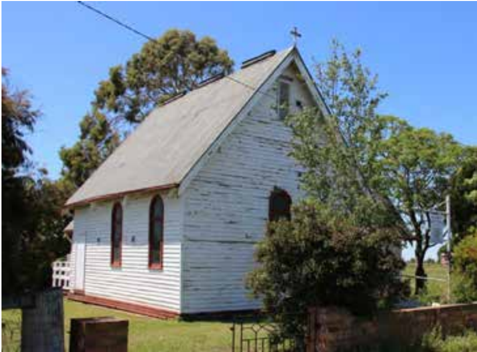
Figure D1. The weatherboard nave has a steep-pitched gabled roof clad in corrugated iron and semicircular-arched windows with coloured leadlight.
