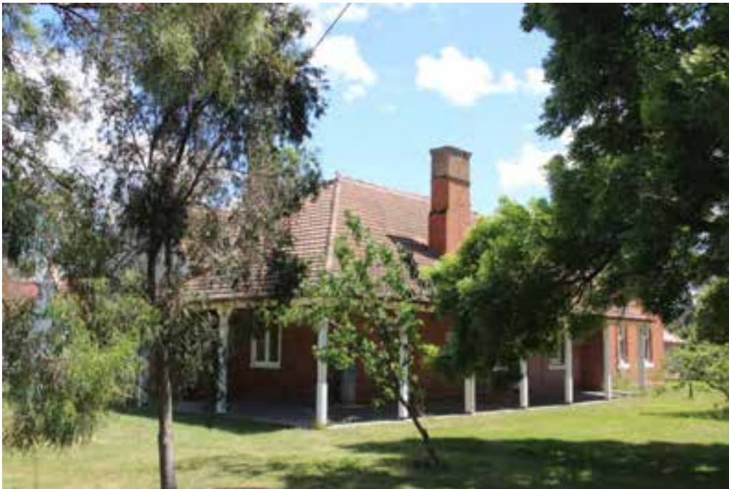
Figure D10. The right side of the façade has a verandah, created by the continuation of the main roofline, which returns on the north elevation. The verandah retains the original timber floor.
