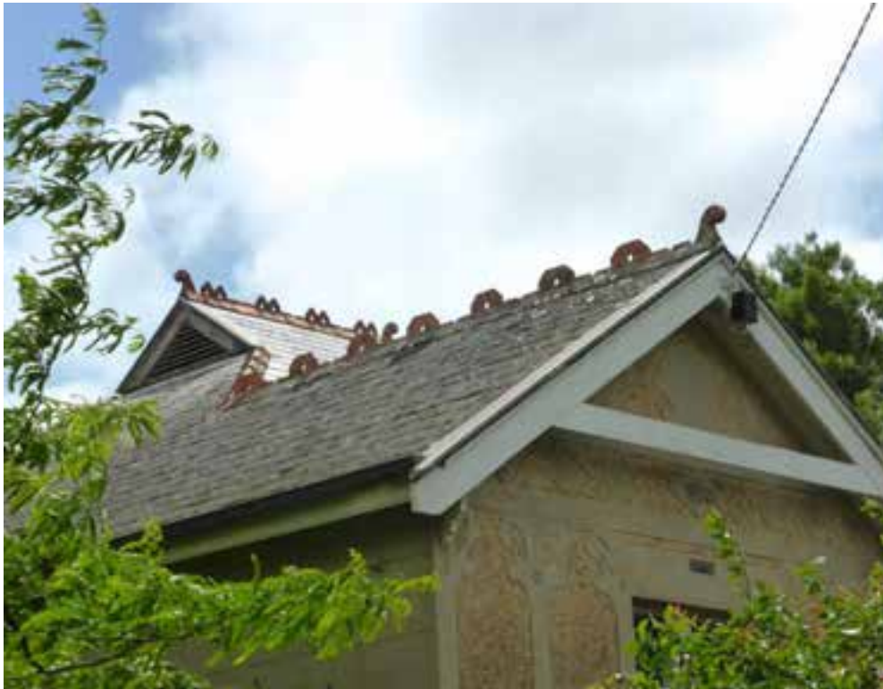
Figure D3. The elaborate hipped and gable roof is clad in slates, with terracotta ridge cresting and finials. The decorative wall pattern can be seen in the gable end.
