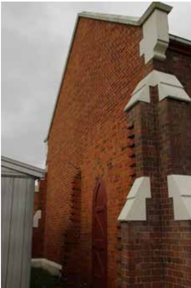
Figure D6. The rear (north) elevation is of red brick. Keyed bricks remain on the right side, that were ready for an extensions that never eventuated. The space in between the keyed bricks has a pointed-arch opening with a timber ledged and framed door.
