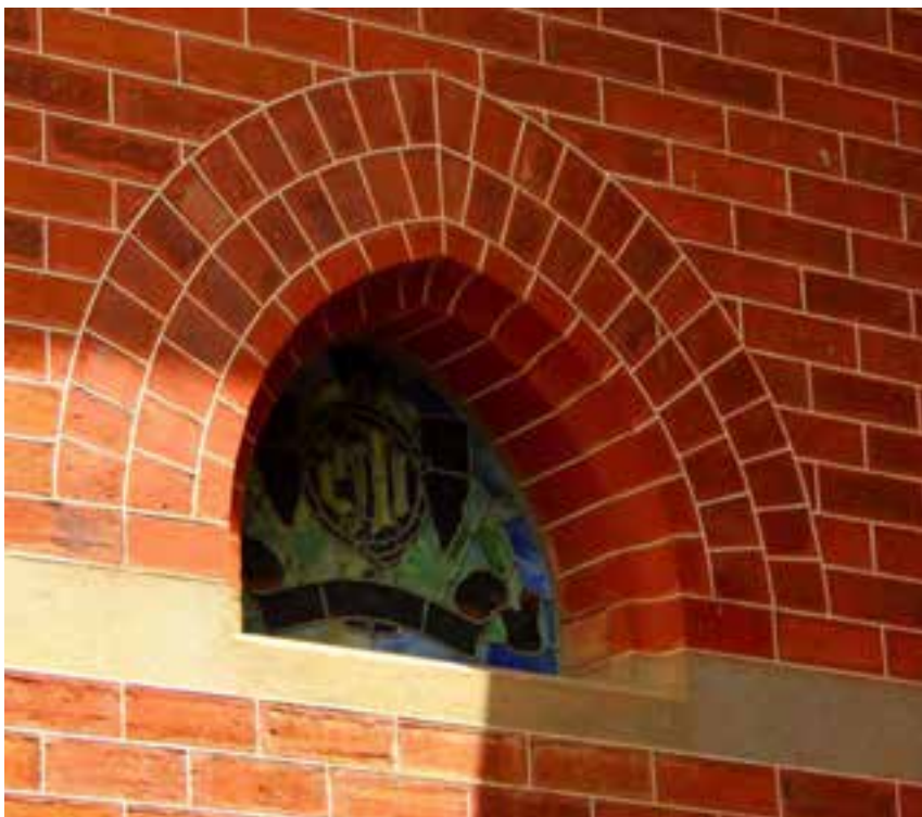
Figure D6. Detail of the exquisite 98 year old brickwork and tuck pointing of the lime mortar, unpainted render and lead lighting, which is all in excellent condition. It should never be painted or treated with any modern sealants. This is testimony to the excellent design, quality of the materials, the builder's skills, and the skills of the craftsmen who created the tuck pointing and lead light by hand.
