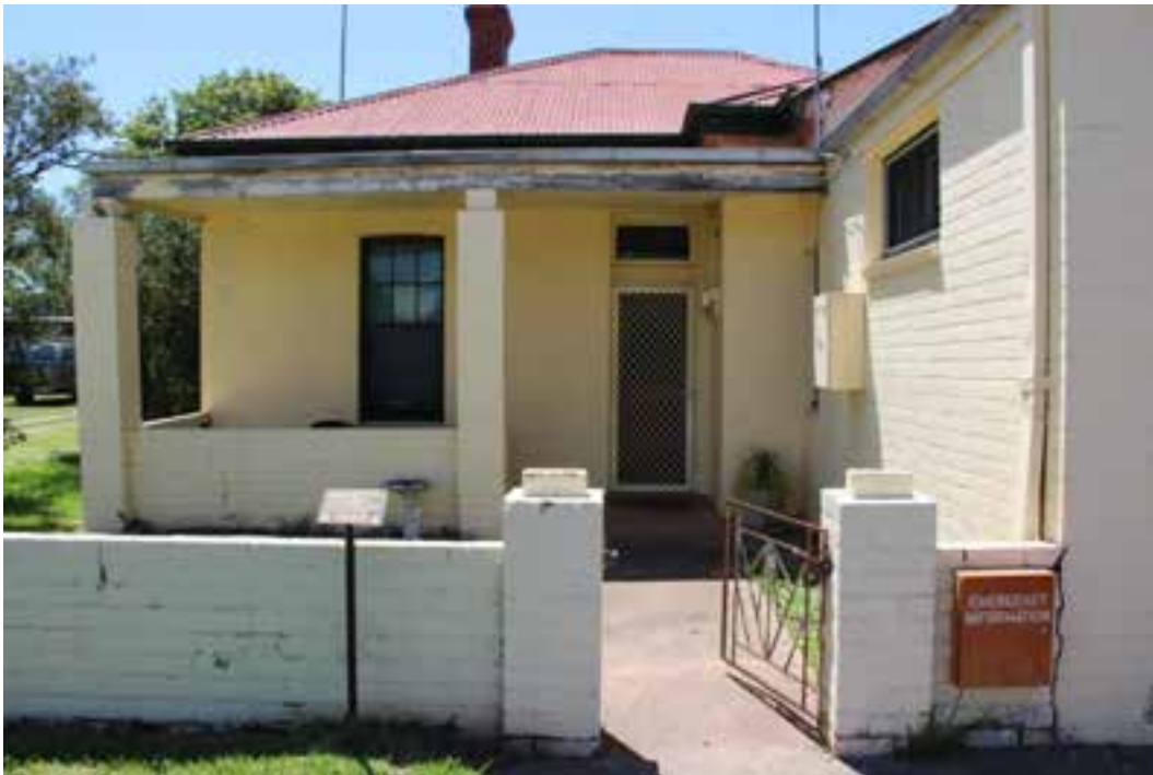
Figure D5. The 1902 building has a projecting gabled-bay to the right of the facade, with a recessed porch to the left, with an entrance door (behind a modern security door) with a highlight, and six-over-six sash window with a segmental-arched opening. A flat-roofed verandah with brick piers and a brick balustrade probably date to the interwar period or later.
