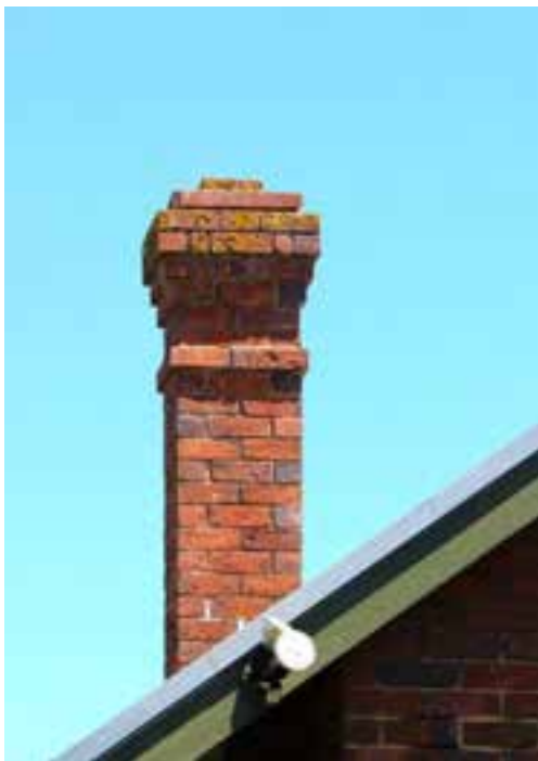
Figure D6. Detail of the corbelled chimney made of the bricks from the Foster family kiln. The bricks and chimneys on other Foster sponsored homes in Boisdale are very similar.
