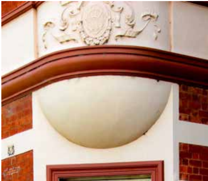
Figure D4. Detail showing the oriel balcony, rendered moulding, flat rendered bands, bank insignia in relief render, decorative wall vent and tuckpointed red brickwork. All the render on this building was originally unpainted and remained that way for about 80 years.
