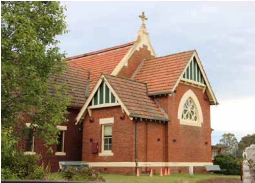
Figure D4. The rear (south) of the church retains the original chancel and two vestry buildings, which project off the chancel to the east and west, all of which continue the detail of the nave. The south elevation of the chancel has a wide pointed-arch opening with a leadlight rose window.
