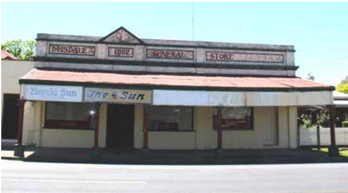
Figure D1. The brick general store has a tall parapet to the facade conceals the roof and has simple Classical mouldings and a pediment above the main entrance. The parapet has the (modern) painted words 'BOISDALE 1907 GENERAL STORE' over remnants of earlier painted words.
