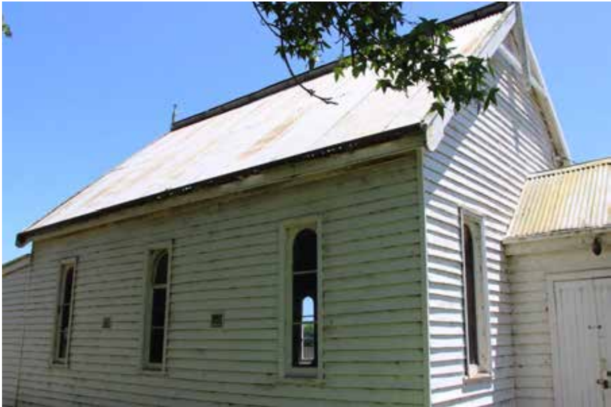
Figure D3. The side elevations comprise three tall windows, with small vents in-between. The windows to the nave have clear glass in three parts; the top portion being a hopper window. The central window has an open hopper in the photo above (not all windows are original). To the rear of the church is the later skillion-roof addition which is not significant.
