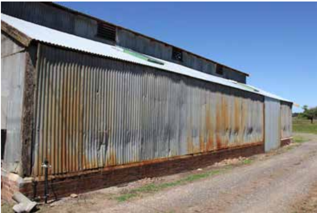
Figure D2. The northern elevation of the stables, with the galvanised corrugated iron walls sitting on the brick plinth, the timber-louvered vents to the clerestory level, and modern skylights to the roof planes below. One large opening is located on this side elevation.
