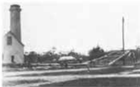
Figure H4. Water tank being erected at Yarram Butter Factory incorrectly dated as 1891 but stack built in 1901. Aylesbury homestead visible in the background. Source. Nicoll, 2008, p. 3
