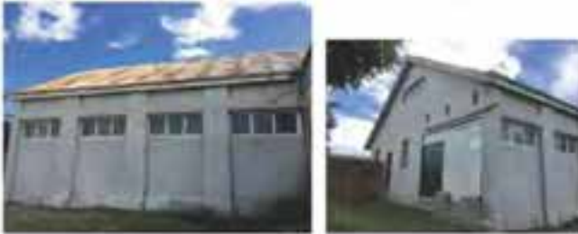
Figure D11. Area G. Left: South elevation of the c1931 factory extension, divided into four bays by pilasters, with highlight windows, and rendered to match the 1931 office building adjacent. Right: The rendered gable end of the single storey extension. The north elevation walls are built of brick with some corrugated iron cladding See Figure D2.
