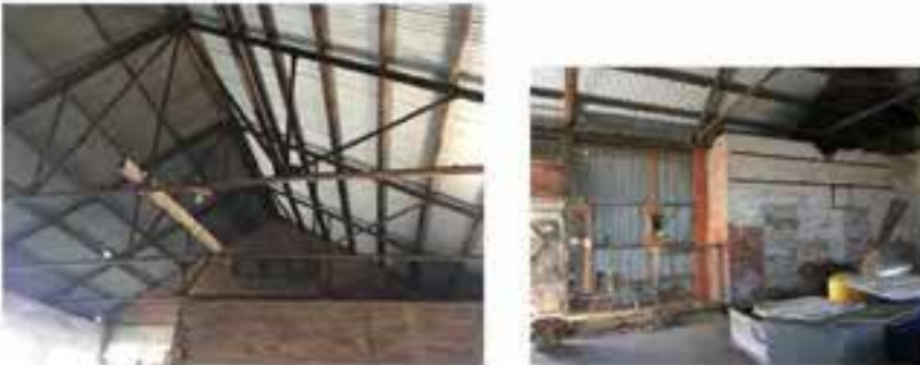
Figure D14. Area G. Left Typical view of the gabled roof of the single storey c1931 factory, with metal roof trusses and galvanised corrugated iron cladding and brown brickwork. Right. View showing red brickwork and corrugated iron walls. The brown brick sections may be earlier remnants of pre 1931 structures.
