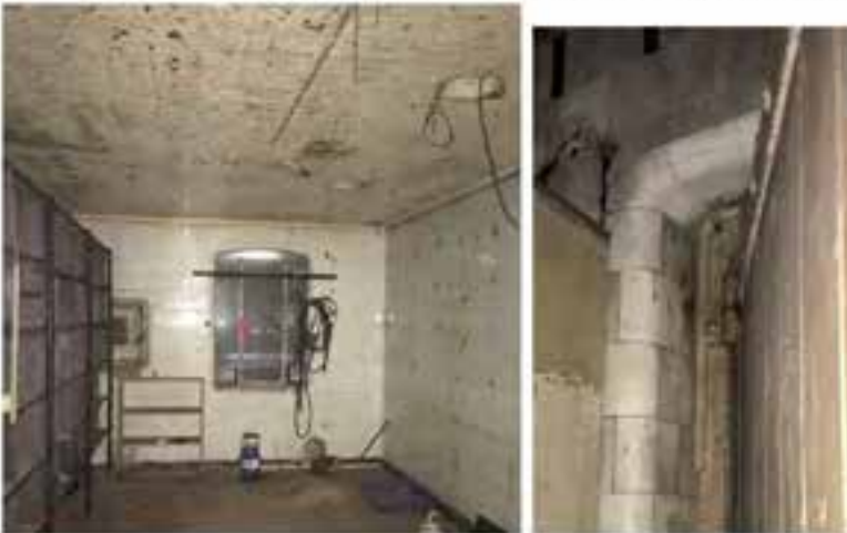
Figure D8. Area C. Looking south to the intact white glazed wall tiles, red-brown hexagon floor tiles, pressed metal ceiling, small hatch, and window and the door opening lined with curved tiles.
