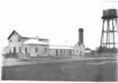
Figure H5. Yarram Butter Factory in 1909 following 1901 additions. Source. Abraham, 1990, 132
