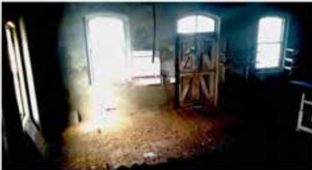
Figure D10. Area J. Looking north, from the loft over area J. Note the intact segmental arched windows, doorway and intact doors. The floor is timber. Source. Andrew Martin 2017.
