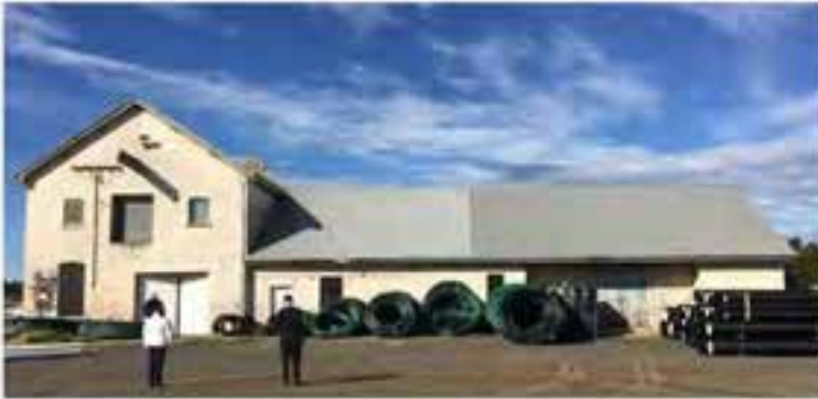
Figure D2. Two storey blue areas A, H. Single storey areas F, G, K. The northern elevation of the existing two storey 1908-09 butter factory (on the left in Figure D2) in which there are three segmentally arched openings with projecting sills dating from 1908-09. Alterations to the two storey section include 'bagging' the red brick wall, enlarging the first floor doorway and inserting a roller door. On the ground floor the double doorway has been enlarged c1931 and double doors inserted. The single storey extension (on the right in Figure D2) is c1931 (and later) is not significant. .
