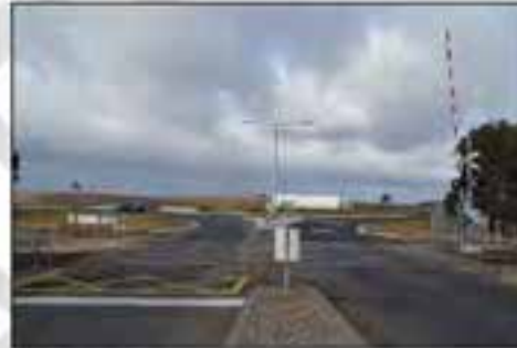
Photograph 9: Hunt Place View South Across Railway Level Crossing to Princes Highway
