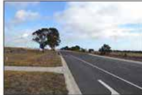
Photograph 2: Princes Highway View West from Reid Drive (Eastbound Carriageway)
