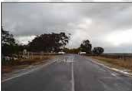
Photograph 12: Williams Drive View North to Railway Level Crossing
