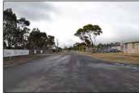
Photograph 7: Hunt Place View East from Riverside Drive
