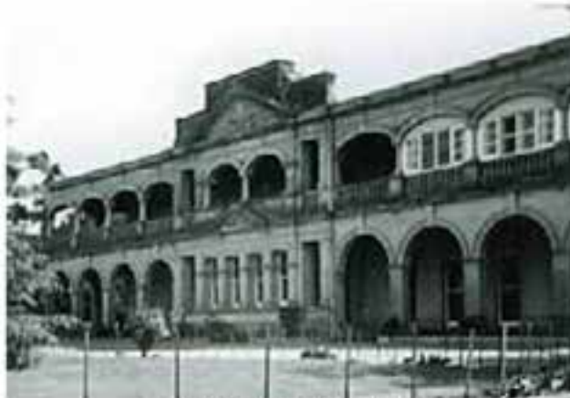
B2969 Kilmany Park Homestead
