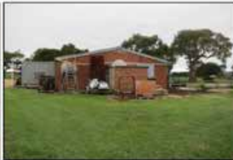
Figure 41 View of the rear (west) elevation of the former water tower. The central arch is concealed behind a modern brick skillion addition. Source: Tretlowan, 2010
