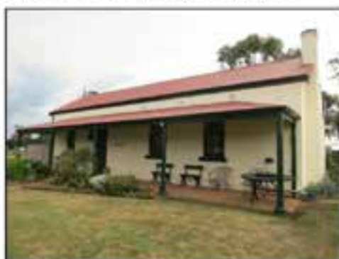
Figure 28 View of the front (south) elevation of the men's quarters. The east end of the building is the earliest, with details indicating it was extended toward the west, c. 1880-81. The door at the left leads to what would have been the original dining room. Source: Tretlowan, 2016
