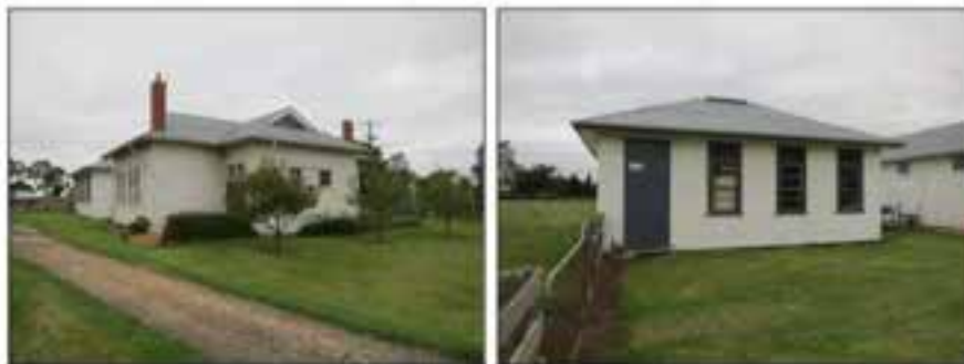
Figures D21 & 22 Source: Trethowan, 2016. p48 School and Sloyd Room.
