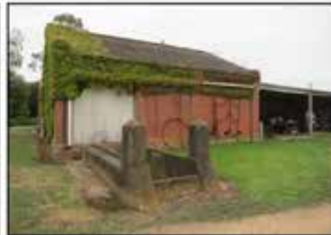
Figure 46 View of the east elevation of the former racing stables. The concrete trough, and skillion roofed shed at left, are later additions. Source: Trefhowan, 2016
