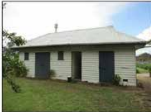
Figure 36 View of the front (south) elevation of the Meat House. The door at the left leads to 'the killing room'. The door at the right leads to a room with an open fire place. Source: Tretlowan, 2016
