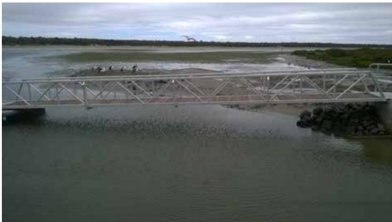
Photo of the gangway and handrails
