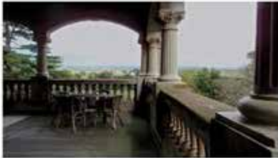
Figure D11. Looking south under the segmental arch, towards Settlement Road, showing the timber floor of the grand first floor balcony, unpainted rendered balustrade and Corinthian composite columns. (2011)
