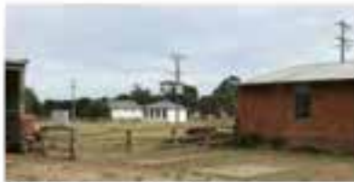
Existing powerline easement across site
