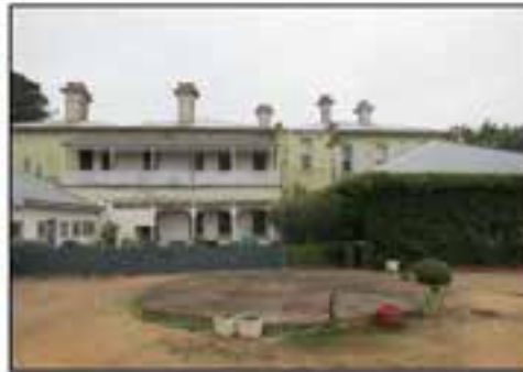
Figure 54 View of the rear (north) elevation of the mansion, looking south. The concrete slab in the foreground replaces the corical cover of the in ground water tank visible in early images. Source: Trefhowan, 2016
