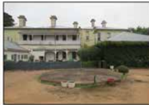
Figure 43 View of the water tank at the rear of the mansion. The concrete cover to the tank is a later addition. Source: Trethowan, 2016
