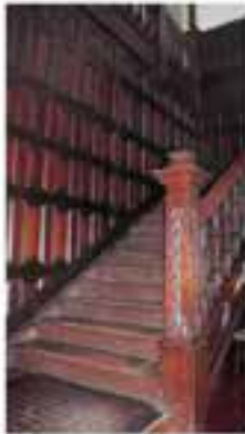
Figure D15. View of the timber staircase with newel post. (2011)
