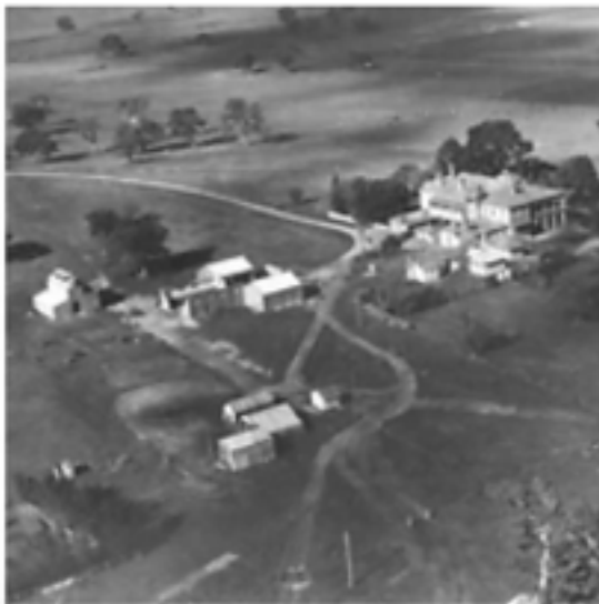
Figure H1. Aerial view c1947 after the 1944 fires, showing the walls of the stables with the roof missing off the rear section of the stables, but the front sections intact. Source.
