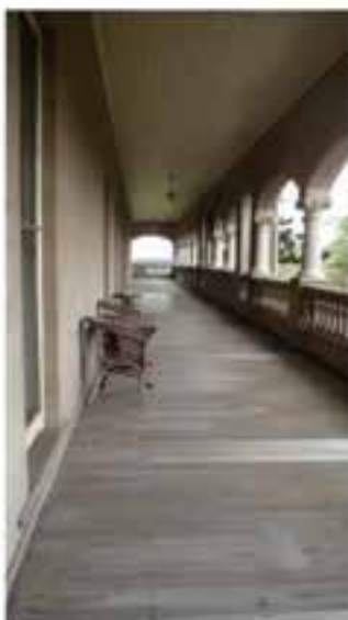
Figure D10. Looking east under the segmental arch, towards the front gates on Settlement Road, showing the unpainted 'ashlar' rendered walls, timber floor of the grand first floor balcony, balustrade and columns. (2011)
