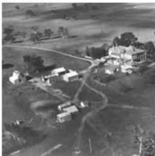
Figure H1. Aerial view c1947 after the 1944 fires, showing the walls of the stables with the roof missing off the rear section of the stables, but the front sections intact. Source: http://www.clan.org.au/perch/resources/kilmanypage-27.5-w640.jpg
