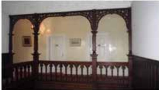
Figure D13. First floor timber balustrade, columns and screen above the stair hall. (2011)
