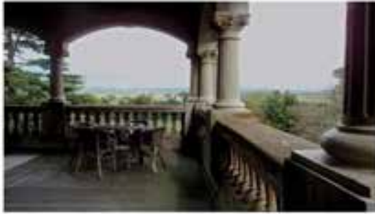
Figure D11. Looking south under the segmental arch, towards Settlement Road, showing the timber floor of the grand first floor balcony, unpainted rendered balustrade and Corinthian composite columns. (2011)
