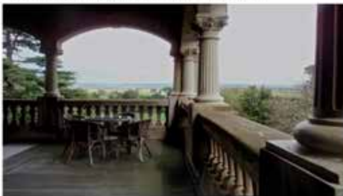
Fig 3. Looking from the upstairs balcony towards the driveway.
