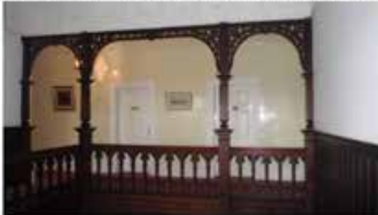
Figure D13. First floor timber balustrade, columns and screen above the stair hall. (2011)
