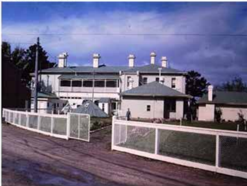
Figure H3. C1947 photo showing the rear elevations of the mansion, (overpainted) including the significant number decorated chimneys, the conical roof over the underground tank, the Meat House to the right. Source: http://www.clan.org.au/homes/vic?s=kilmany-park-house-presbyterian-home-for-boys .
