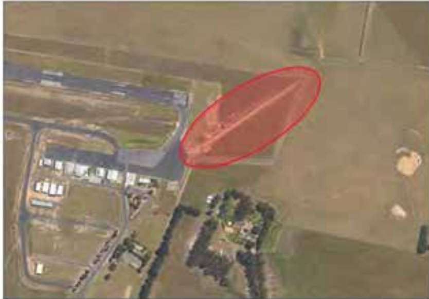
Figure 23: Open stormwater drain
