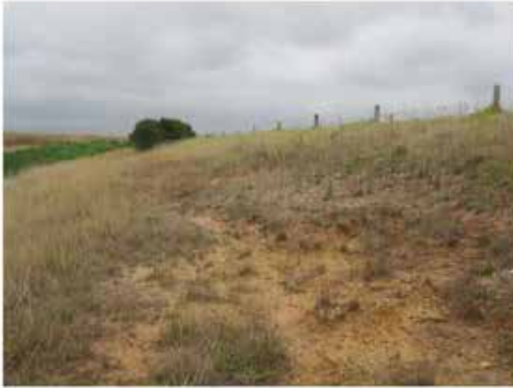
Figure 6: Erosion Embankment (in foreground)
