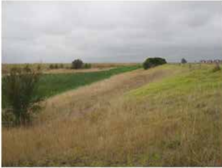
Figure 4: Bushes on Embankment
