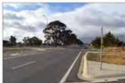
Photograph 1: Princes Highway View East from Reid Drive (Westbound Carriageway)
