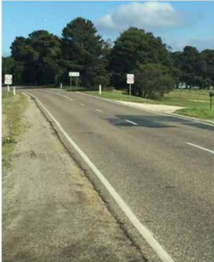
Photograph 4: View looking west along Rosedale-Longford Road from the intersection with Brennans Road
